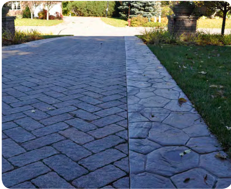
Figure 3.5: Paver driveway with stamped concrete border.
