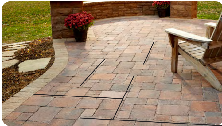
Figure 4.4: A bad example of a random paver pattern with straight lines longer than four feet.
