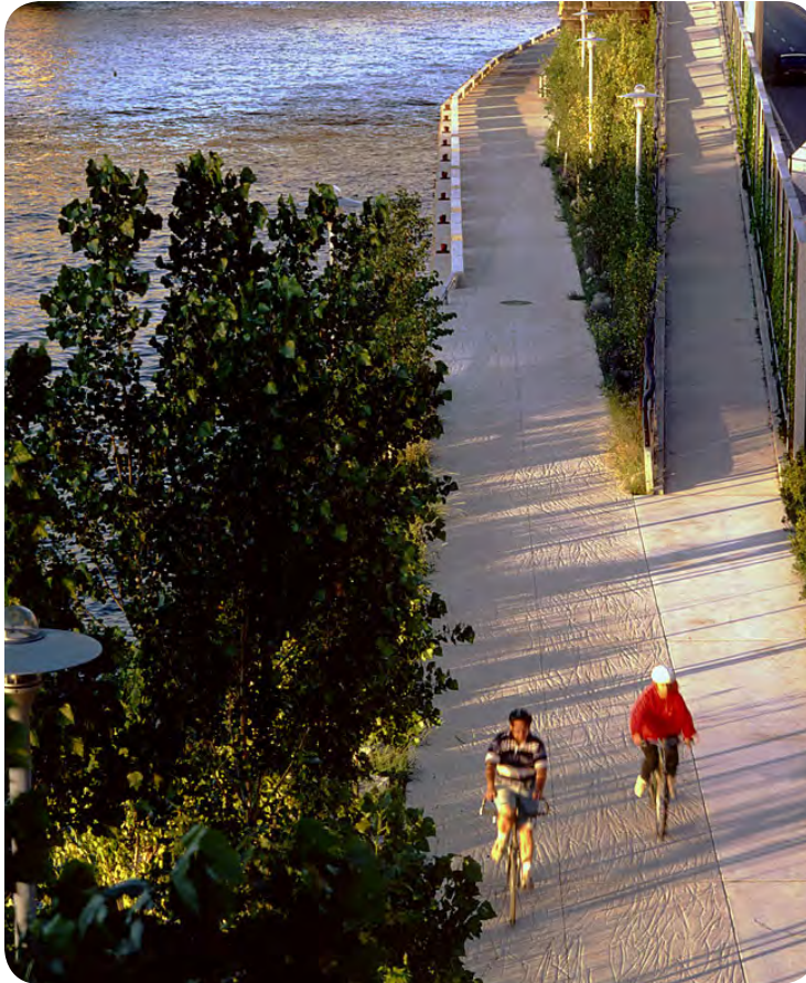
Figure 1.11: Reed inlaid concrete sidewalk, smooth enough to bike on, yet detailed enough to notice.
