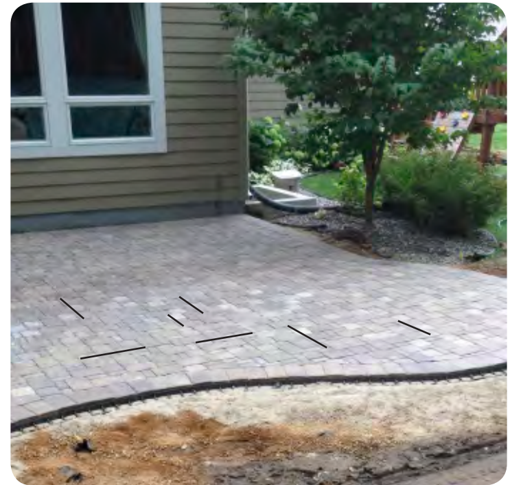
Figure 4.5: A good example of a random paver pattern with no straight lines longer than four feet.
