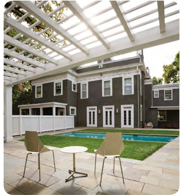
Figure 1.6: The pergola creates human scale and matches the geometry of the fence.
