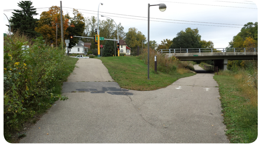
Figure 2.3: Example of existing bike trail conditions. (Photo Credit: Josh Wildt, October 2013)
