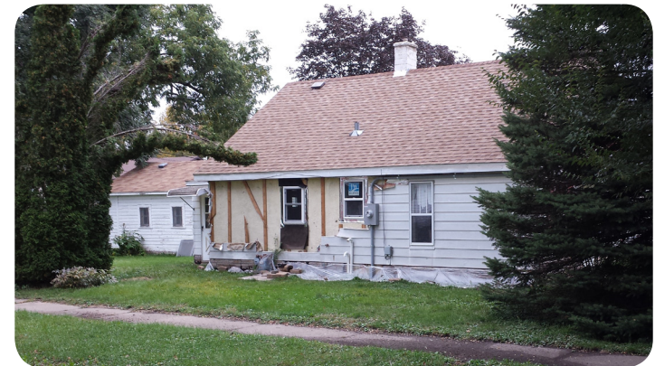
Figure 3.3: House under repair in Washington Neighborhood (Photo Credit: Josh Wildt)
