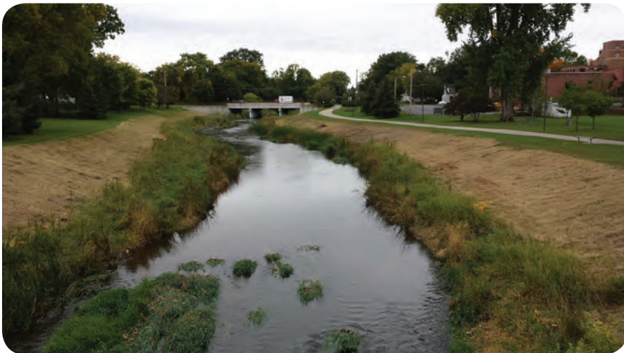
Above: Engineered channels that form a majority of the Creek.
