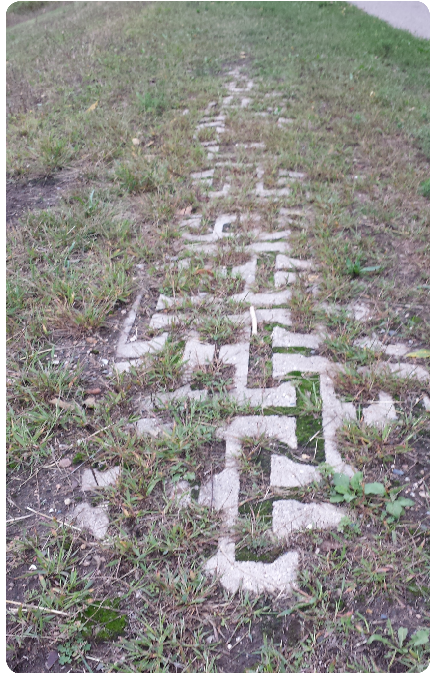
Figure 3.9: Another example of a riprap bank. (Photo Credit: Josh Wildt)
