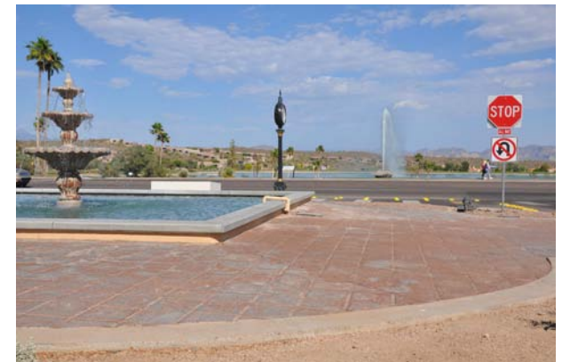
Image showing the intersection between the Avenue of the Fountains and Saguaro Boulevard.
