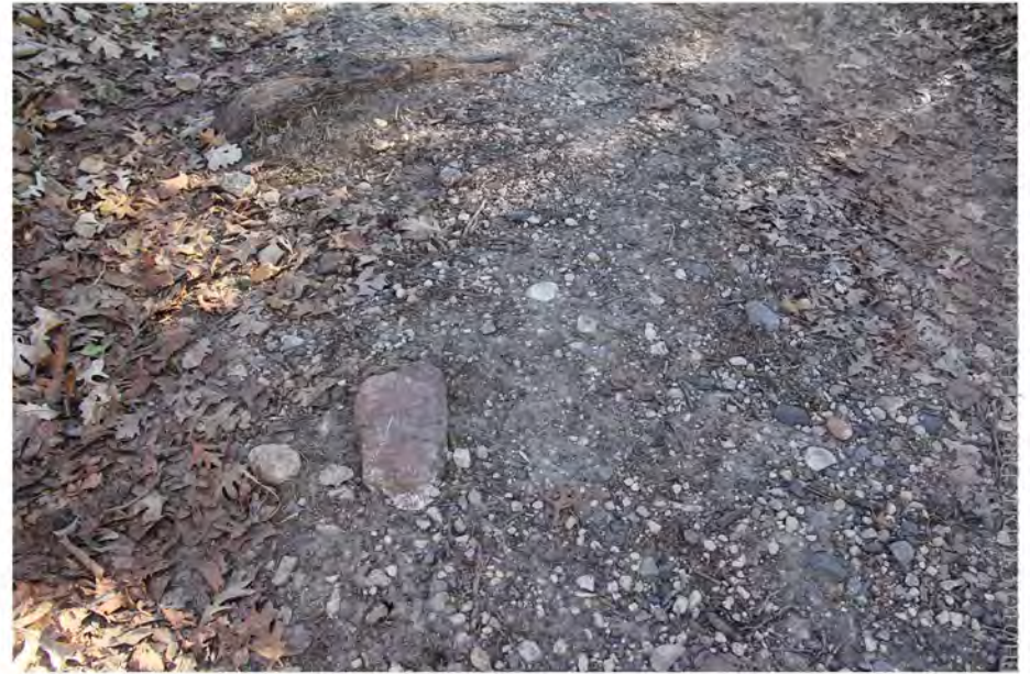
3.18 Exposed Boulders and Roots Caused By Erosion
