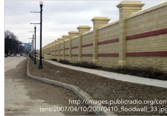
This image depicts a floodwall in Grand Forks North Dakota, illustrating the physical disconnect between urban environment and the river.
