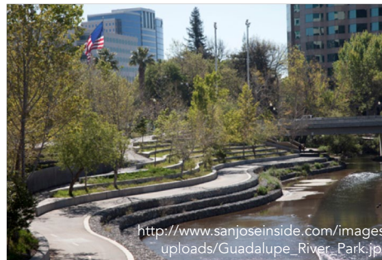
This image shows the riverbanks along the Guadalupe River, demonstrating an alternative flood control measure.
