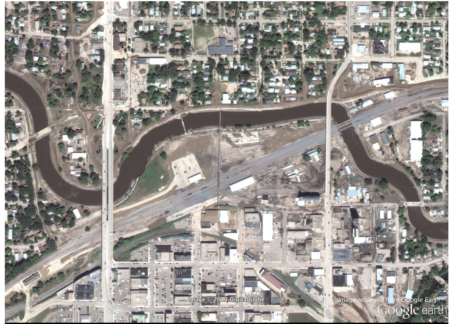
Site After Flood - July 26th, 2011
