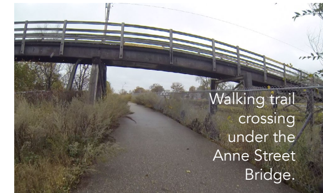
Damaged walking trail as a result of 2011 flood.
