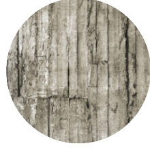
Striated Concrete Interior Structural Walls
