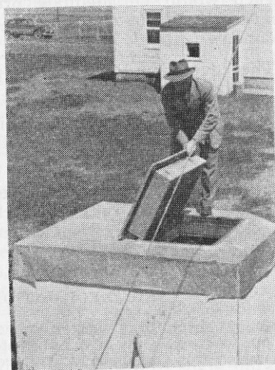
Fig. 6—Sheep barn pump house. (Manhole opens directly over pump.)
