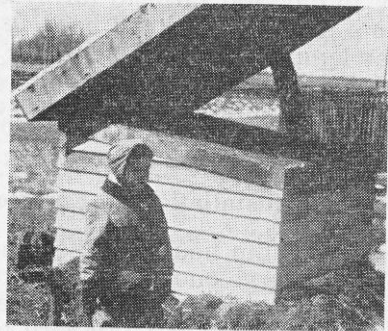
Fig. 4—Smith pump house with cover raised. (This is an unsafe method of supporting the cover.)
