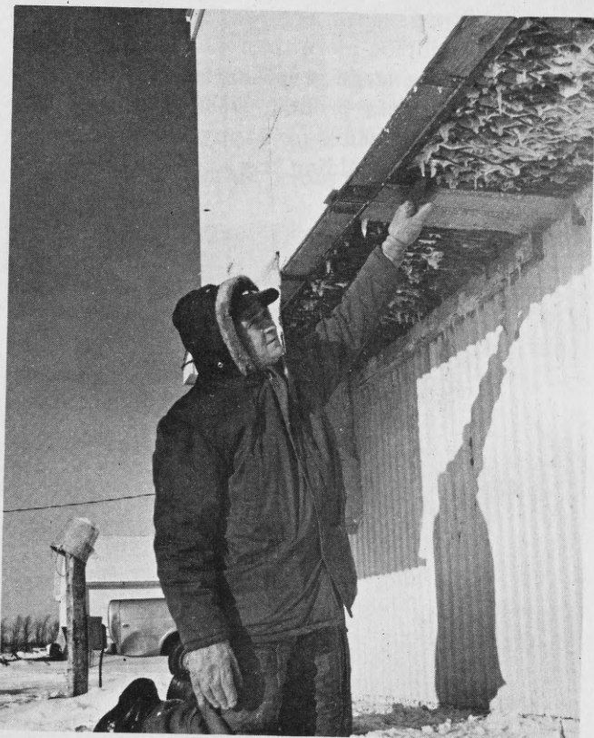
Agricultural engineer Richard Witz examines the heat exchanger unit at the confinement beef barn. In this heat exchanger, a layer of rocks is heated by exhausted warm air, and this heat is then used to warm incoming ventilation air when the flow is reversed.
