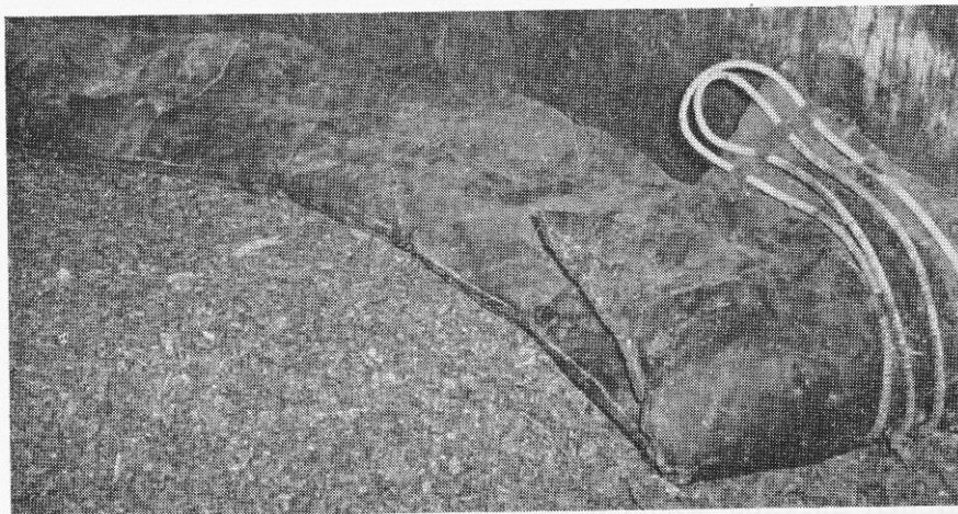
FIGURE 3.— The insulated blanket with the lead covered wires enclosed with flexible conduit and attached to the blanket.
