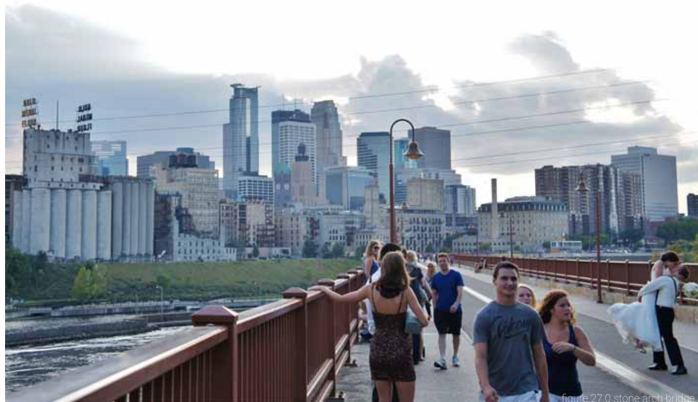
figure 27.0 stone arch bridge
