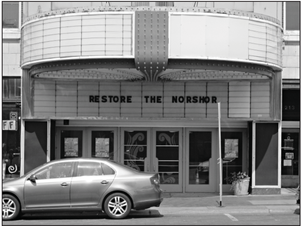
Figure 02 | Nor Shor Marquee Today
