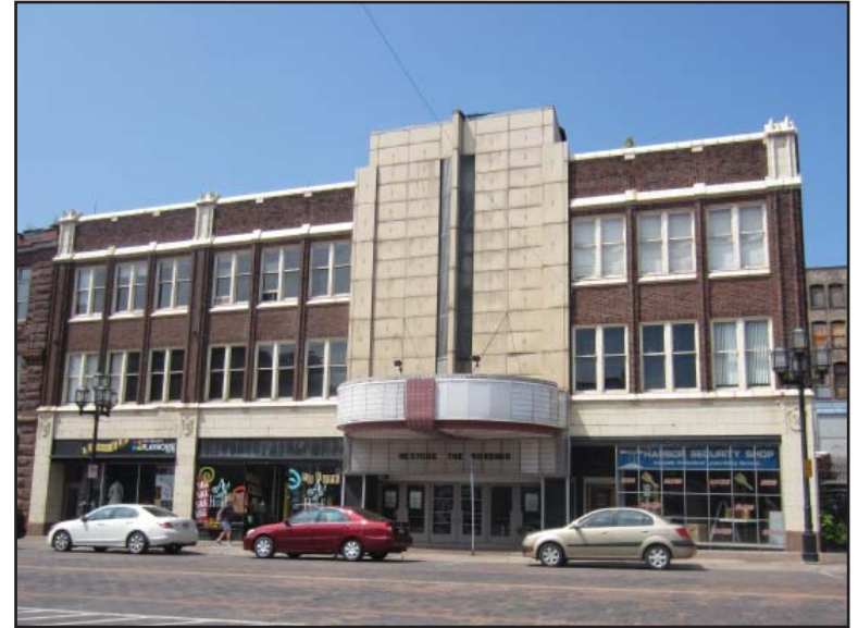
Figure 52 | Nor Shor southeast facing elevation | Duluth, MN
