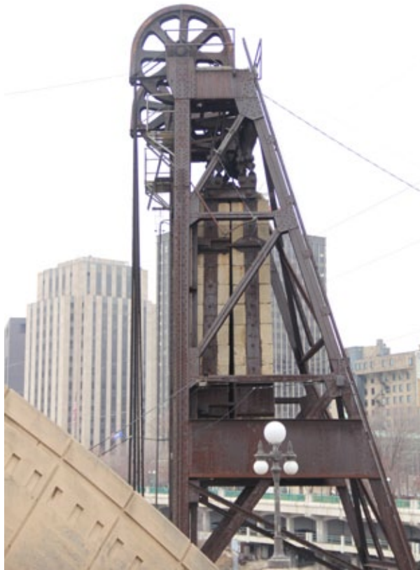
train bridge infrastructure
