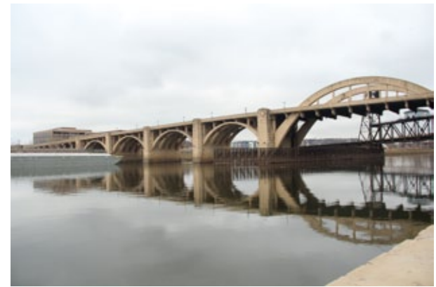
on site, Robert St. Bridge from docking pier
