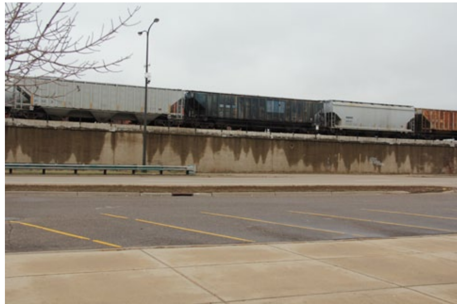
from parking lot on site, facing elevated rail wall
