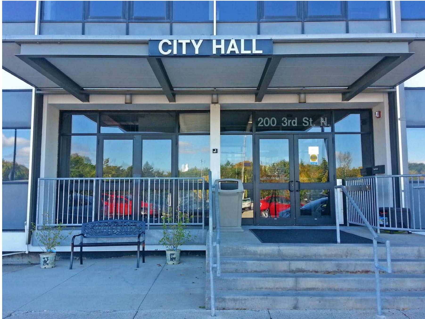
EXISTING CITY HALL BUILDING TO BE DEMOLISHED.
