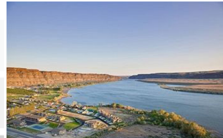
Figure 2.3 Image of Site
