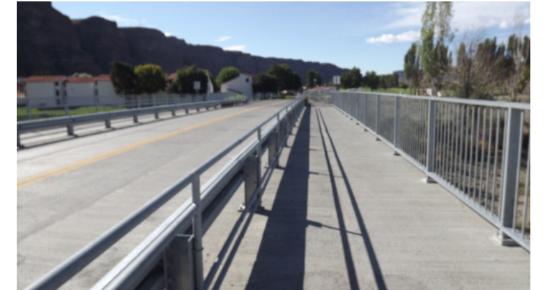
Figure 10.14 Crescent Bar Rd & Sidewalk
