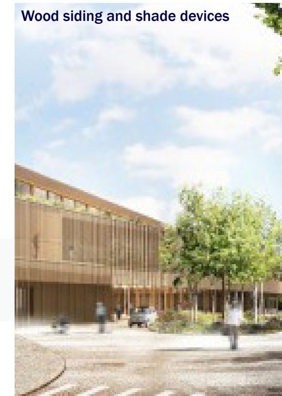
Figure 6.3 Children's Hospital Zurich
