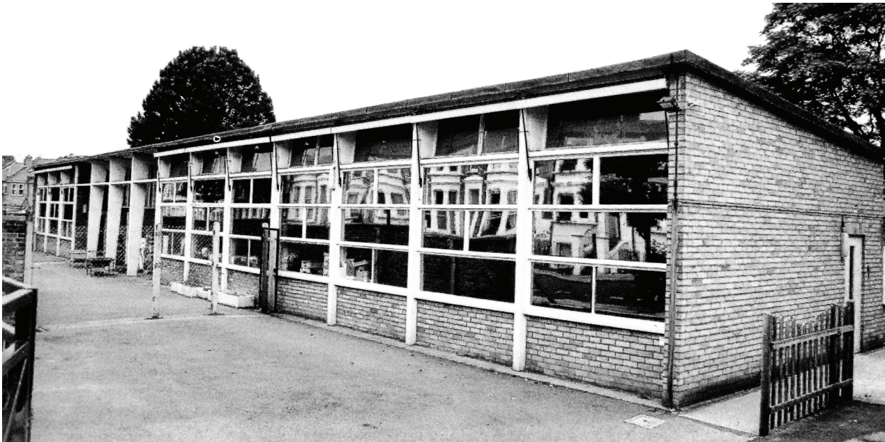
Figure 64. Impington Village College.
