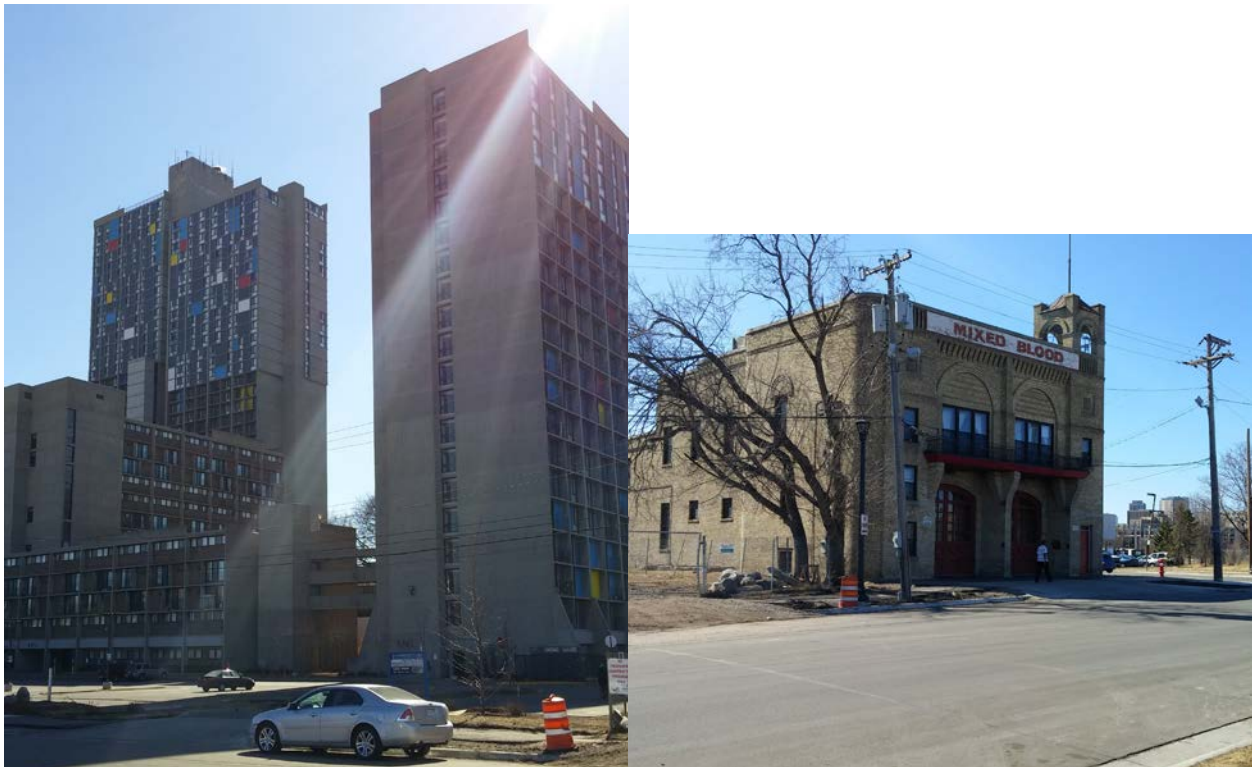
Figures 3.31 [site pictures south]
