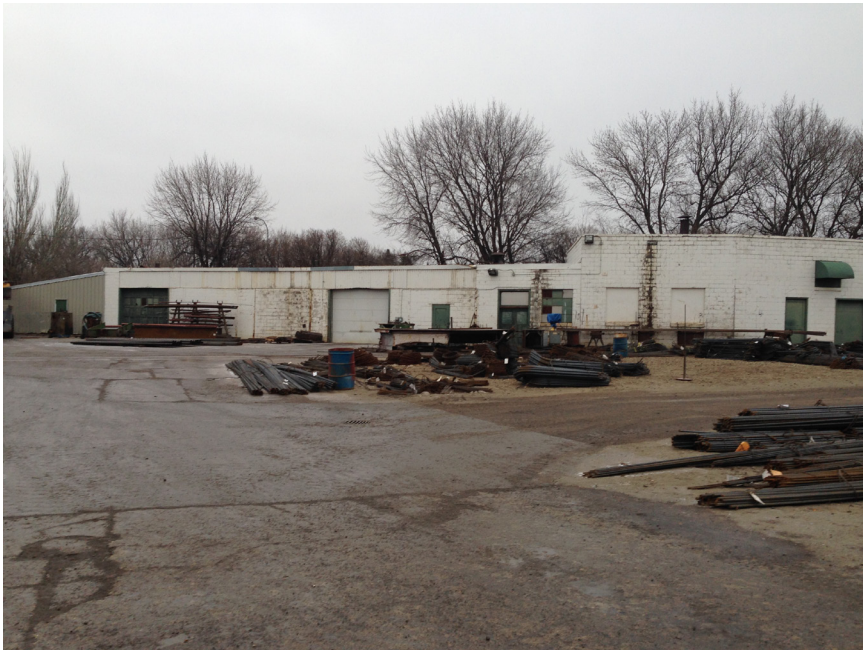
Figure 67 Storage Building, (Author)
