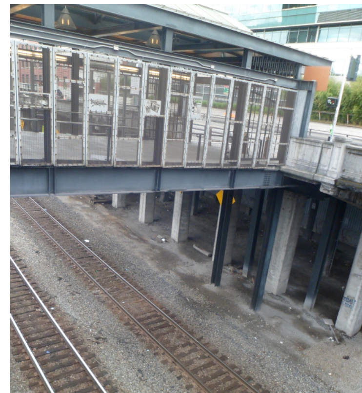
2nd Level Walkway
