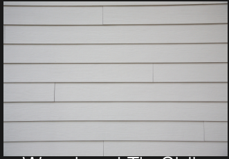
Wood and Tin Siding
