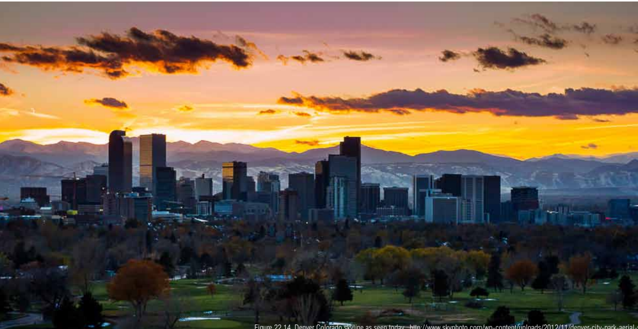
Figure 22.14 Denver Colorado skyline as seen today. http://www.skyphoto.com/wp-content/uploads/2012/11/denver-city-park-aerial-s
