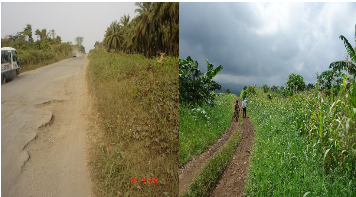
Figure 5. Some poor roads conditions in Fako Division.
