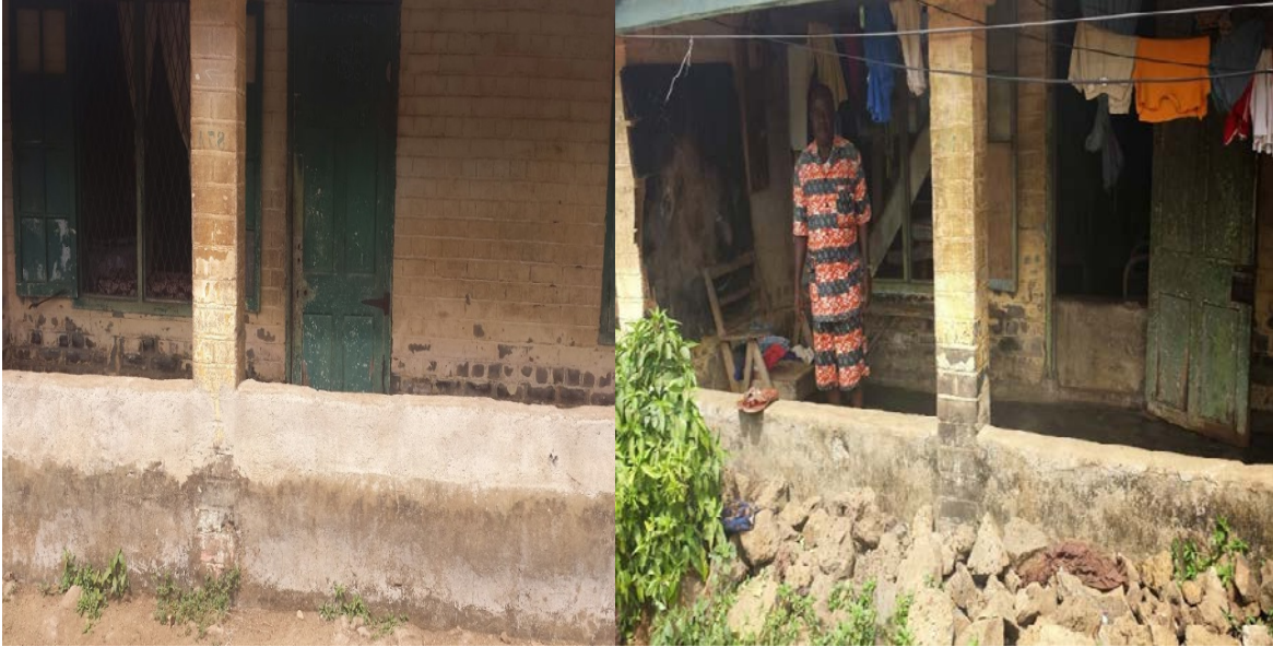
Figure 6. Flood-prevention walls in Clarks Quarters Limbe
