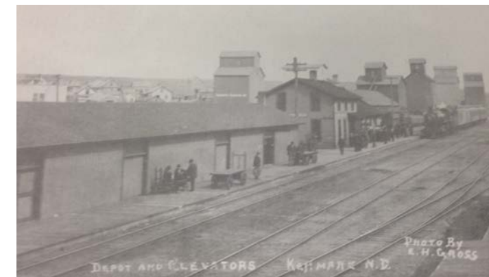
Figure 63.1 - Depot and Elevators, South of Irvin
