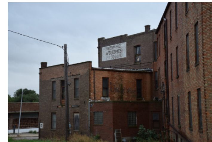
Figure 81.1 - Irvin Hotel North Facades
