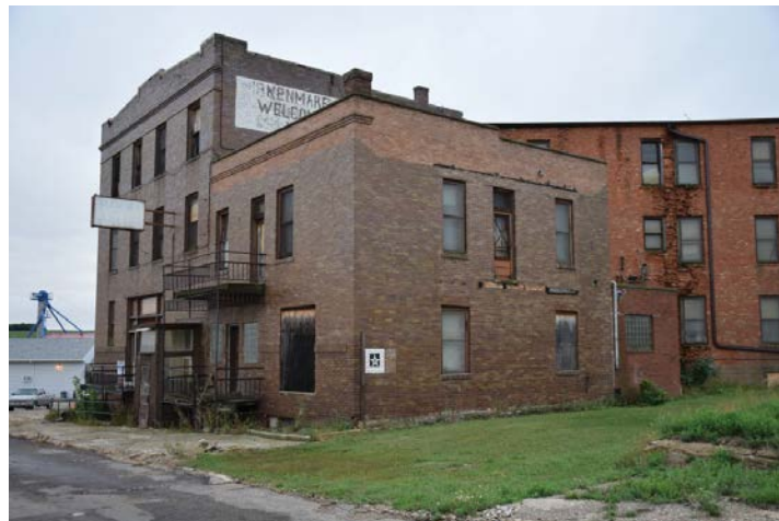
Figure 48.2 - North and East facades
