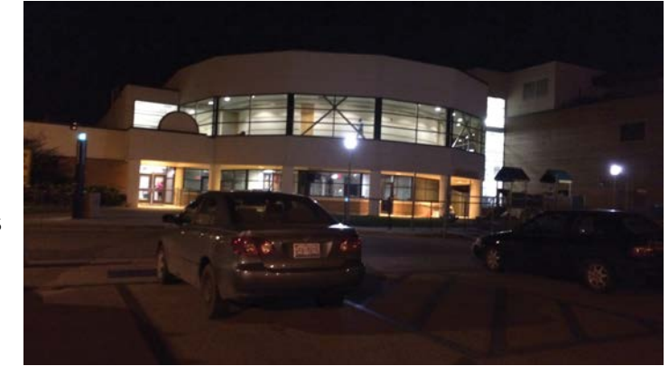
Figure 31.1 - North View at Night
