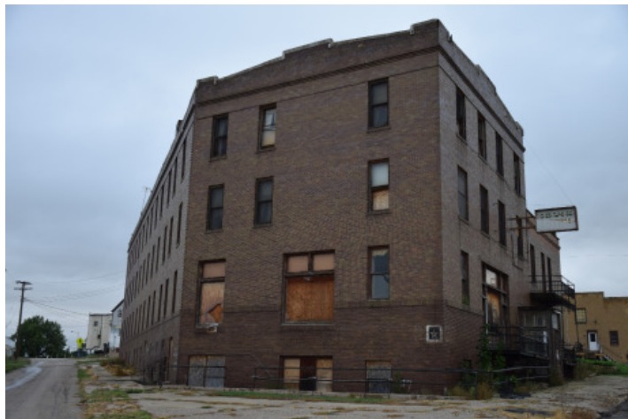
Figure 80.1 - Irvin Hotel East and South Facade
