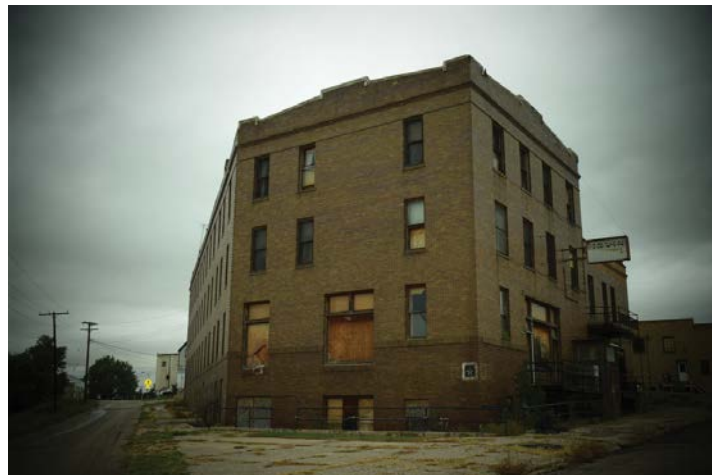
Figure 48.3 - South and East facades
