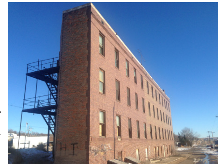
Figure 79.1 - Irvin Hotel West and South Facade
