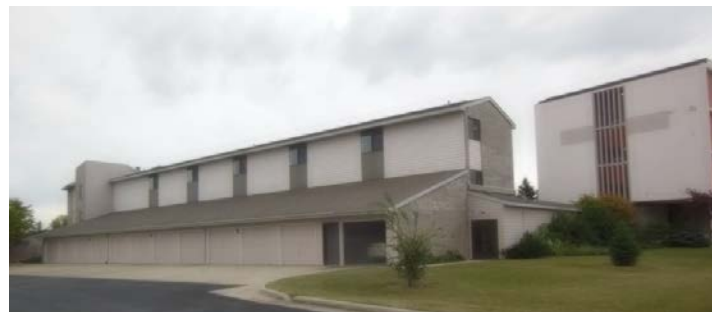
Figure 18.1 - Looking South towards Riverview Place
