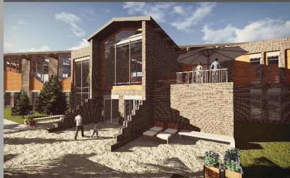
Side Entrance (east)
