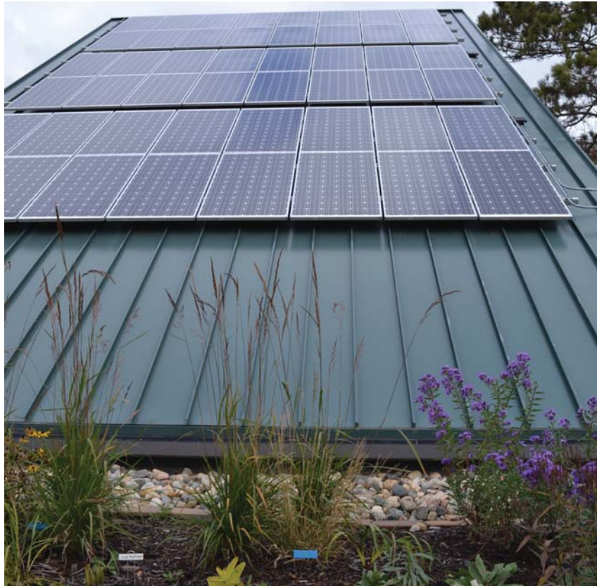
Figure 6 - Tamarac Wildlife Refuge Visitor Center Roof
