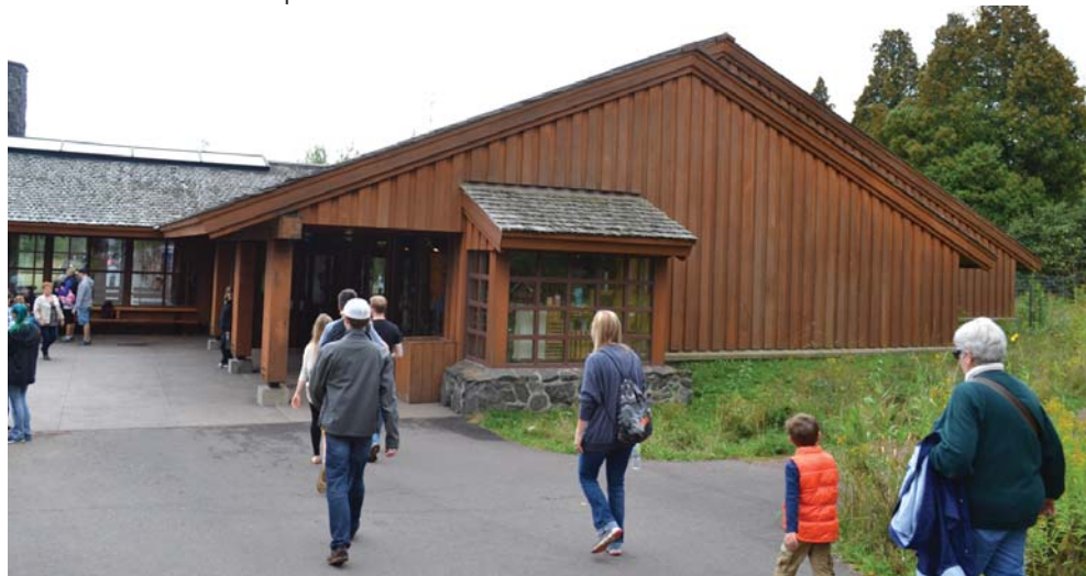
Figure 18 - Gooseberry Falls Visitor Center Exterior Experience
