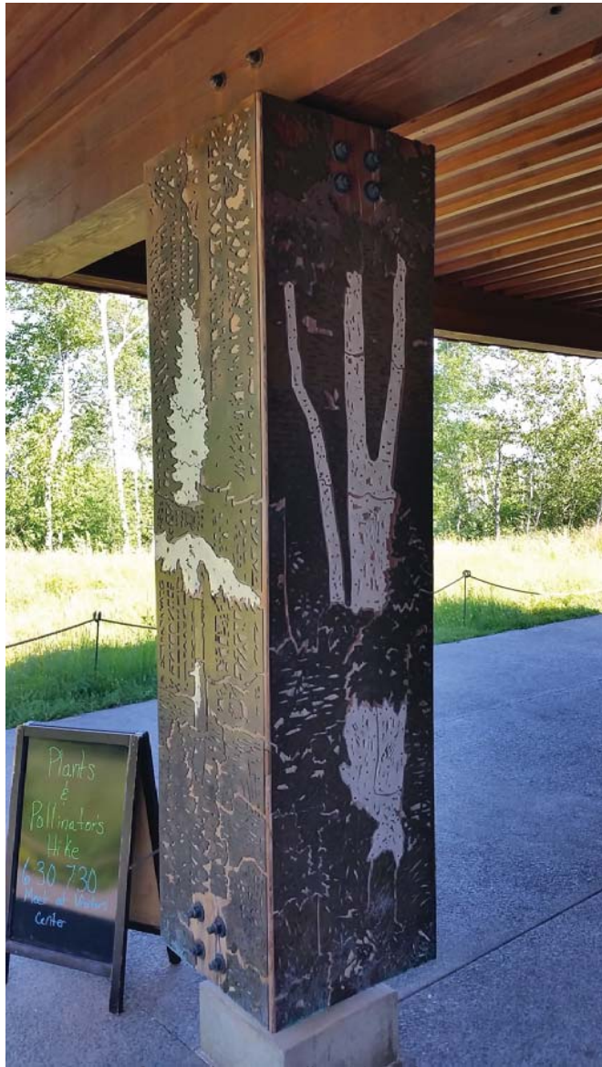
Figure 19 - Gooseberry Falls Visitor Center Exterior Construction
