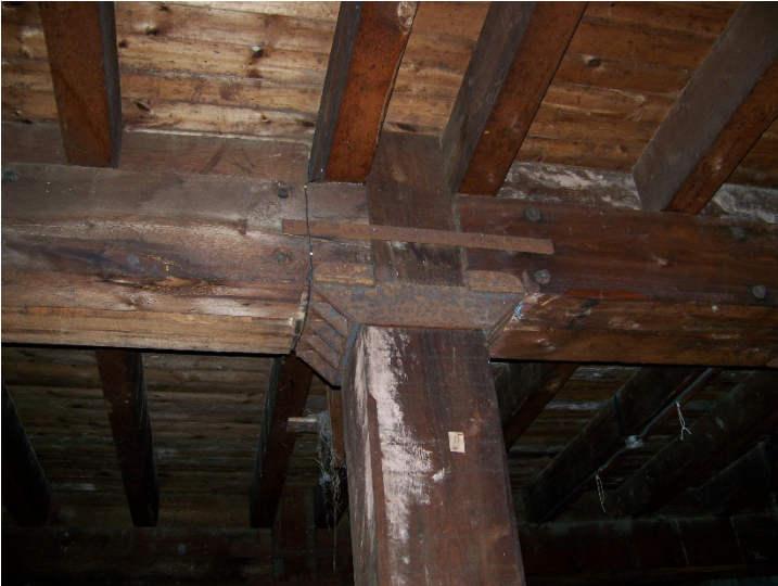
Structural beam and column connection
