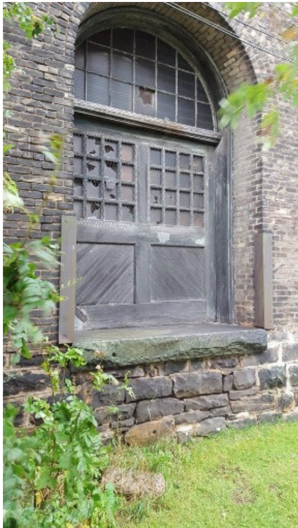
Loading doors on East side
