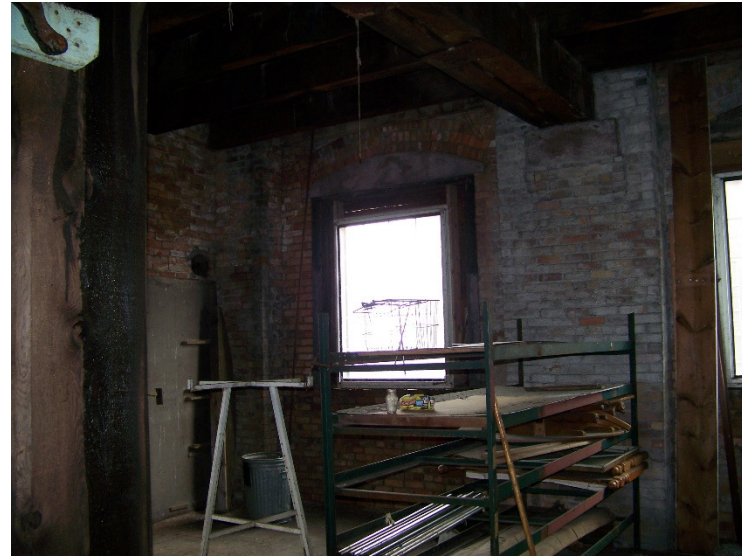
Window on exterior wall
