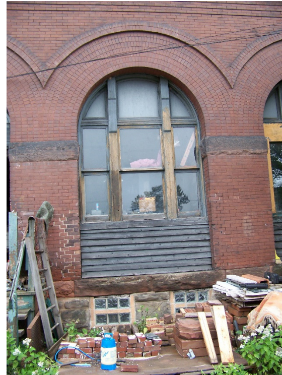
First floor window on west side
