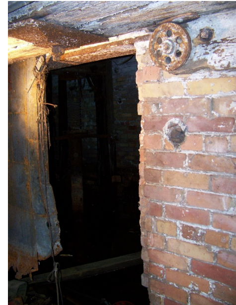
Basement elevator doors
