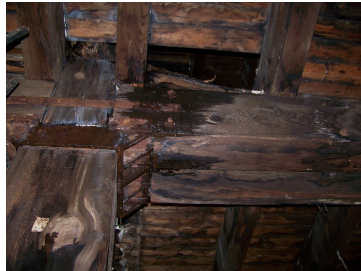
Connection of timber structure
