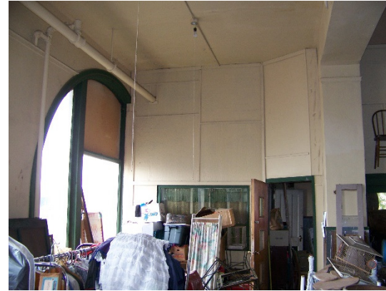
Interior of south side
