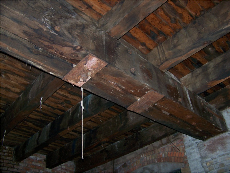
Structural timber beam
