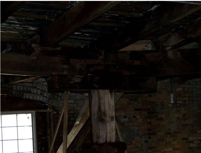
Water damaged structure
