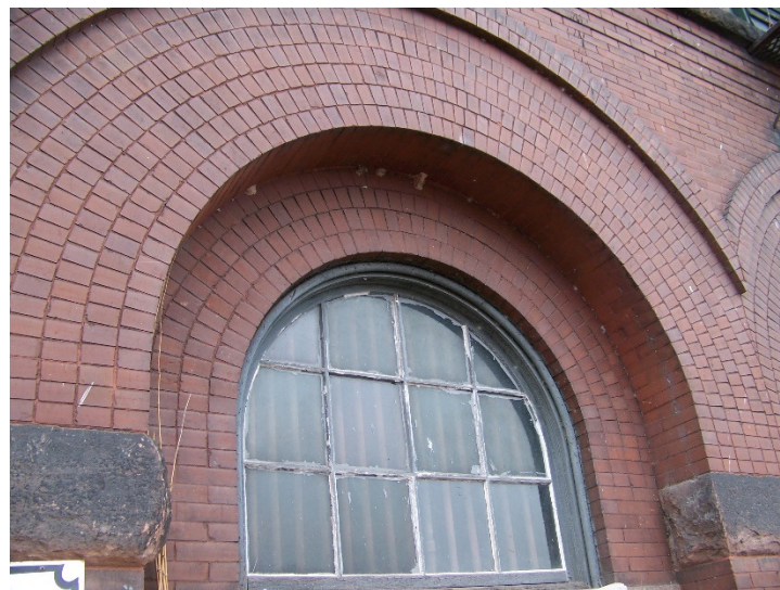
Arch on South side of building
