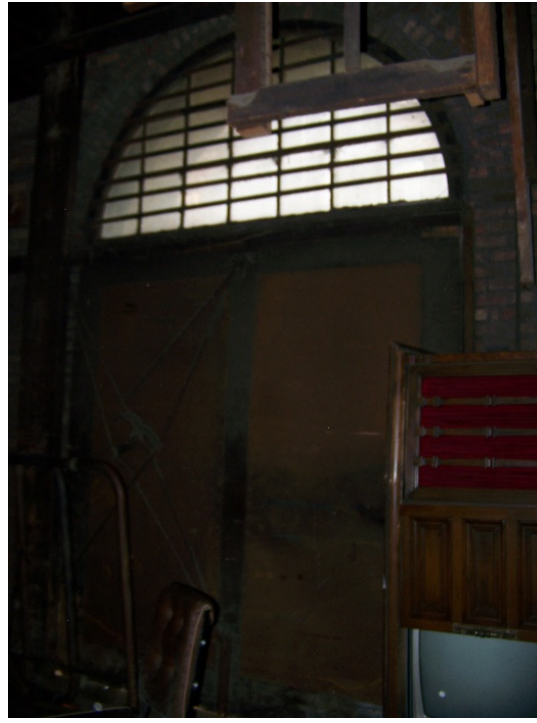
Inside of loading doors
