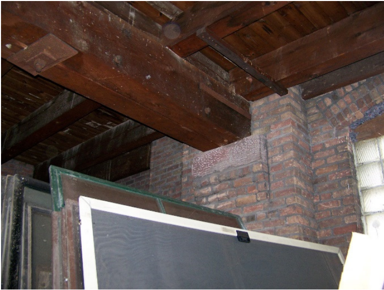
Timber beam meeting exterior wall
