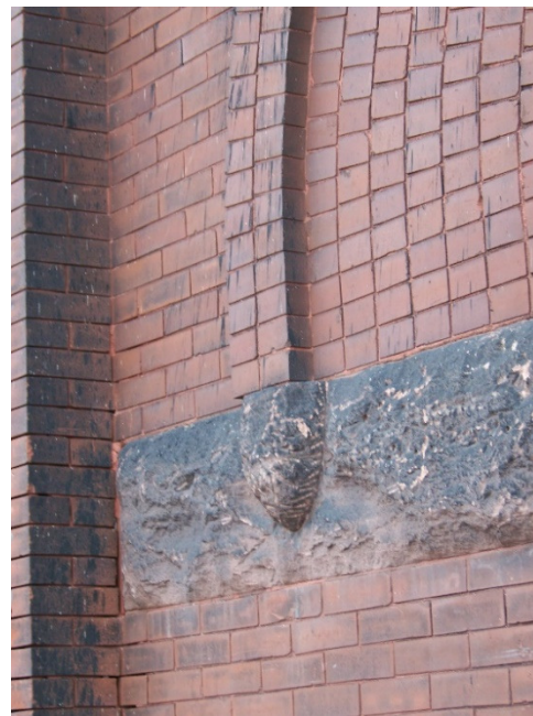
Masonry Detail on South side of building
