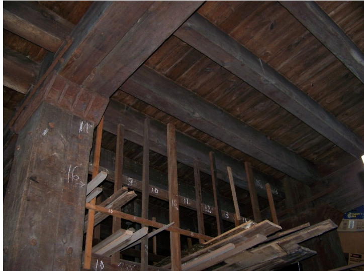
Structural Decking under floor
