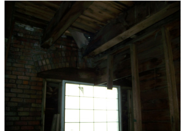
Result of water damage at exterior wall
