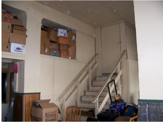
Existing office area
