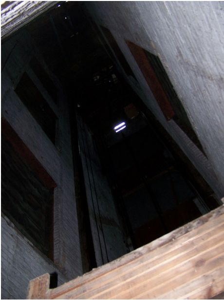
Existing elevator shaft
