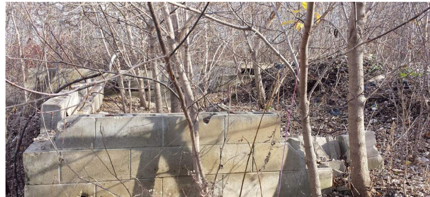
Figure 36 | Image of the existing original foundation for the farmhouse
