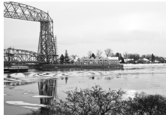
figure 5 | canal park + lift bridge
