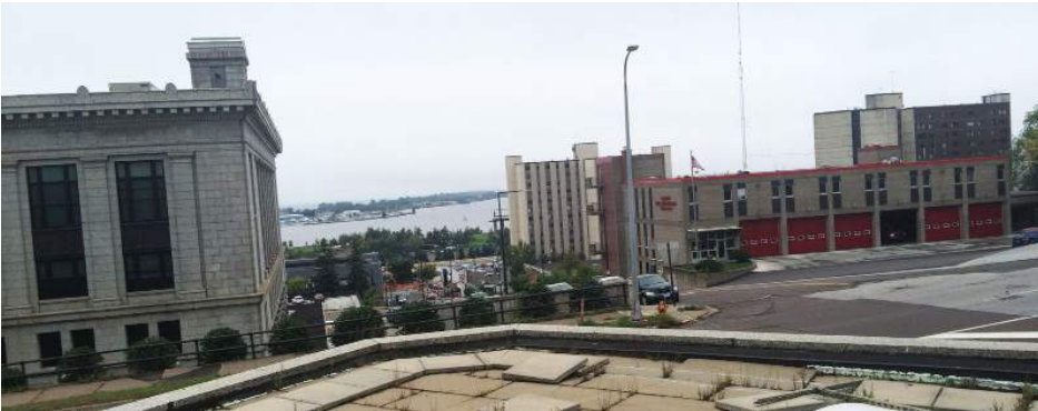
figure 66 | annex rooftop view
