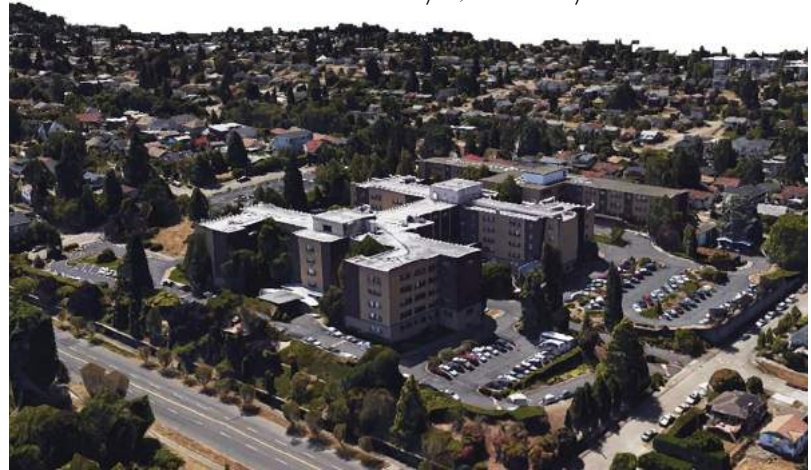
figure 17 | pmsv aerial view
