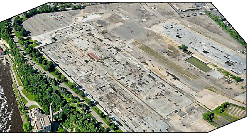
Demolition completed summer 2013
