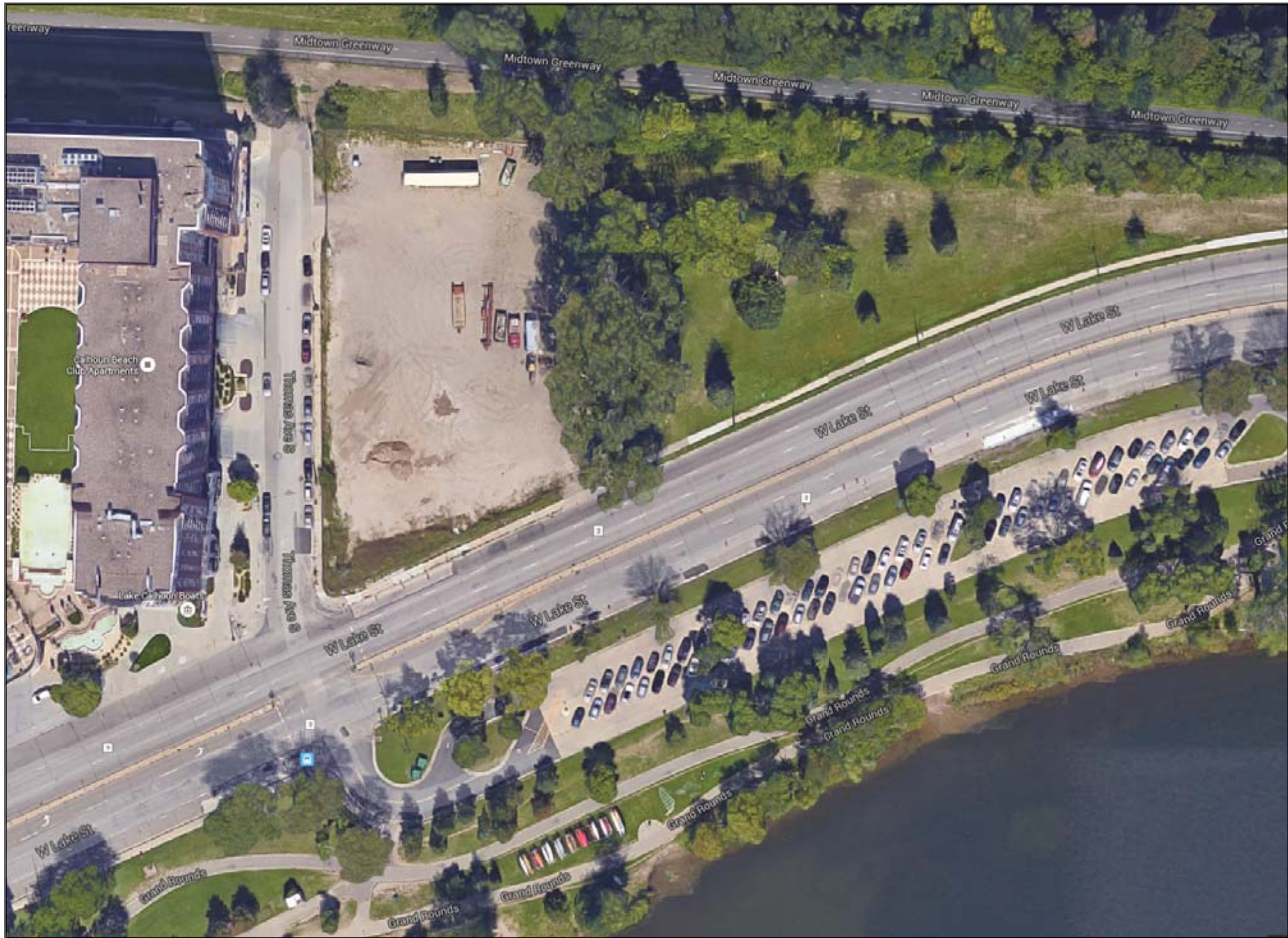
Ariel photo showing site character
