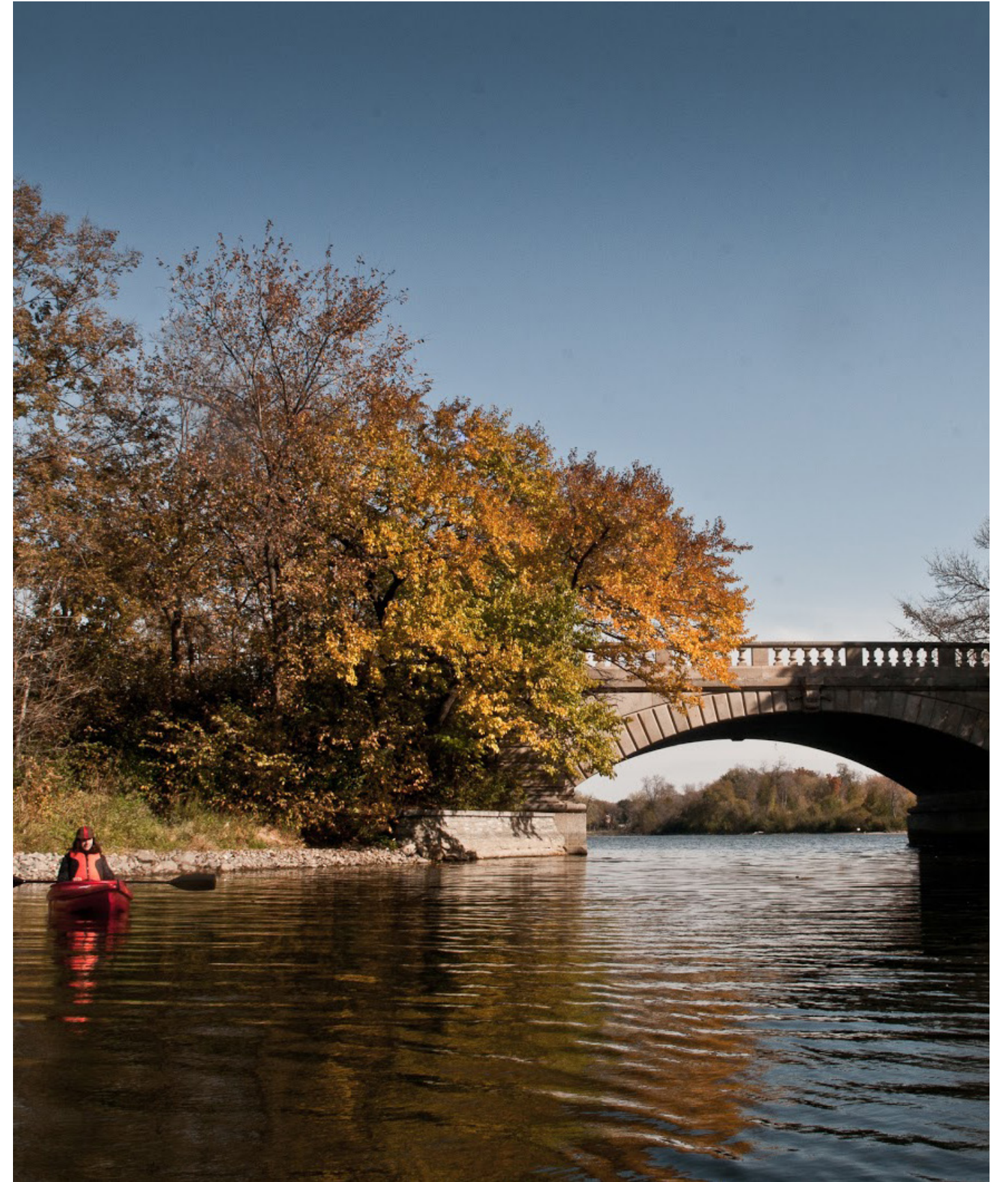
Fig.19: West Lake of the Isles bridge
