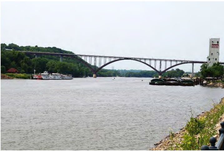
Figure 64: Looking west of the site at the Smith Ave. S. Bridge
