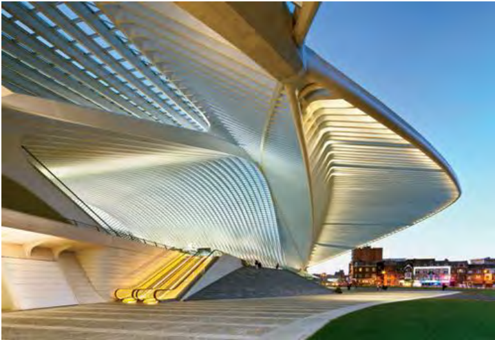
Figure 15: Liege-Guillemins TGV Railway Station Exterior (1). http://archrecord.construction.com/projects/bts/archives/transportation/10_TGV_Railway_Station/default.asp?bts=TR
