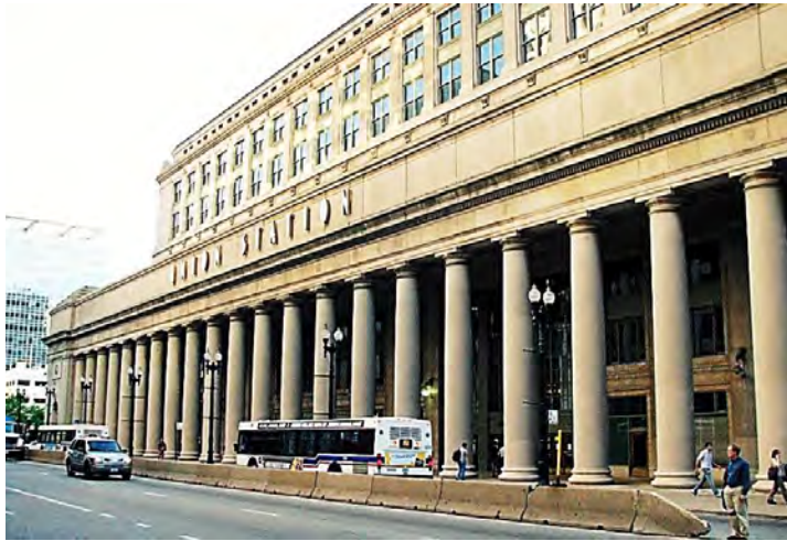
Figure 10: Chicago Union Station.
