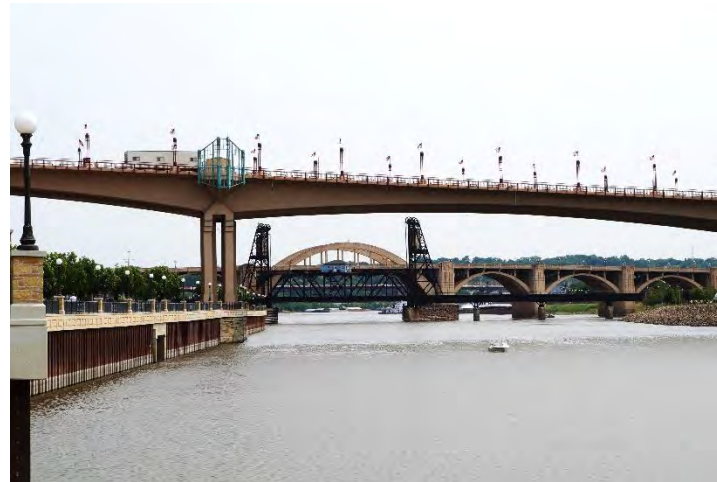
Figure 63: Looking east of the site underneath Wabasha Bridge
