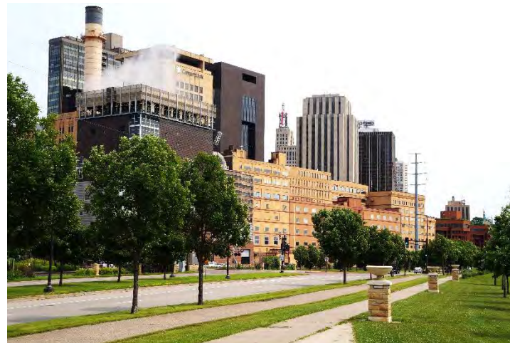
Figure 56: West Publishing buildings and downtown St. Paul, MN
