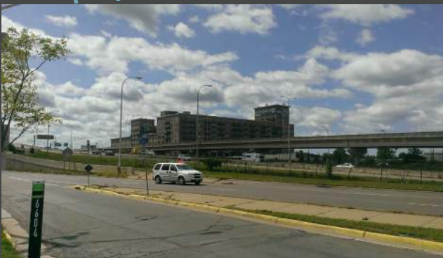
Figure 75 - Picture of west side of site
