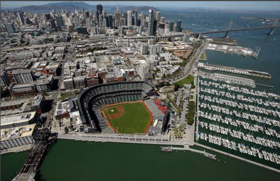
Figure 04 - San Francisco Giants AT&T Stadium, a good example of stadium design integration into its site
