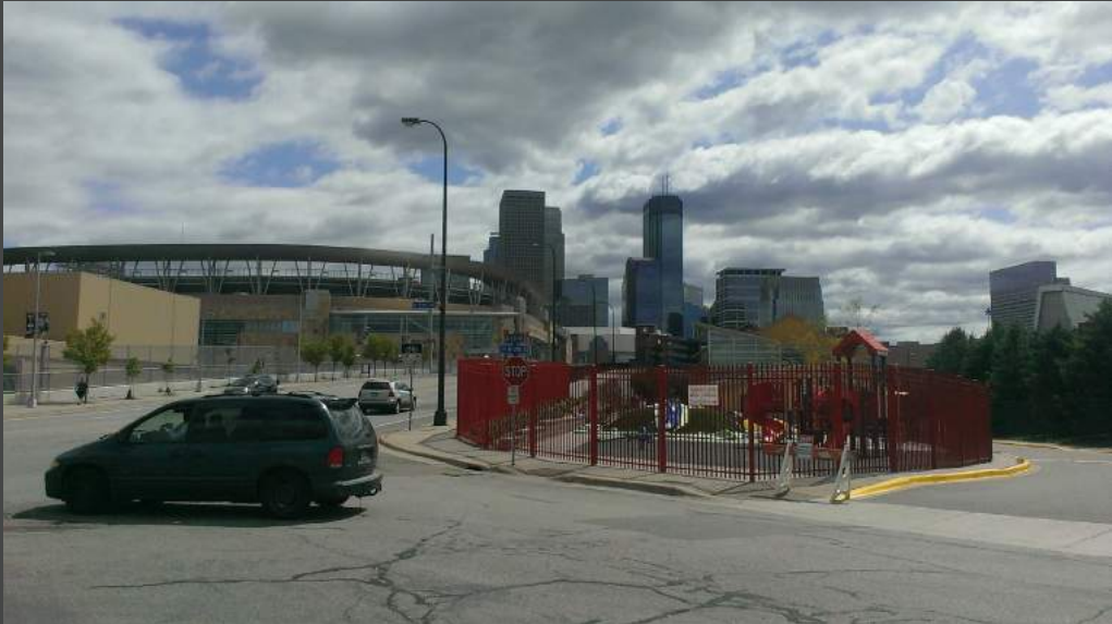
Figure 52 - West approach to Target Field on N 7th St
