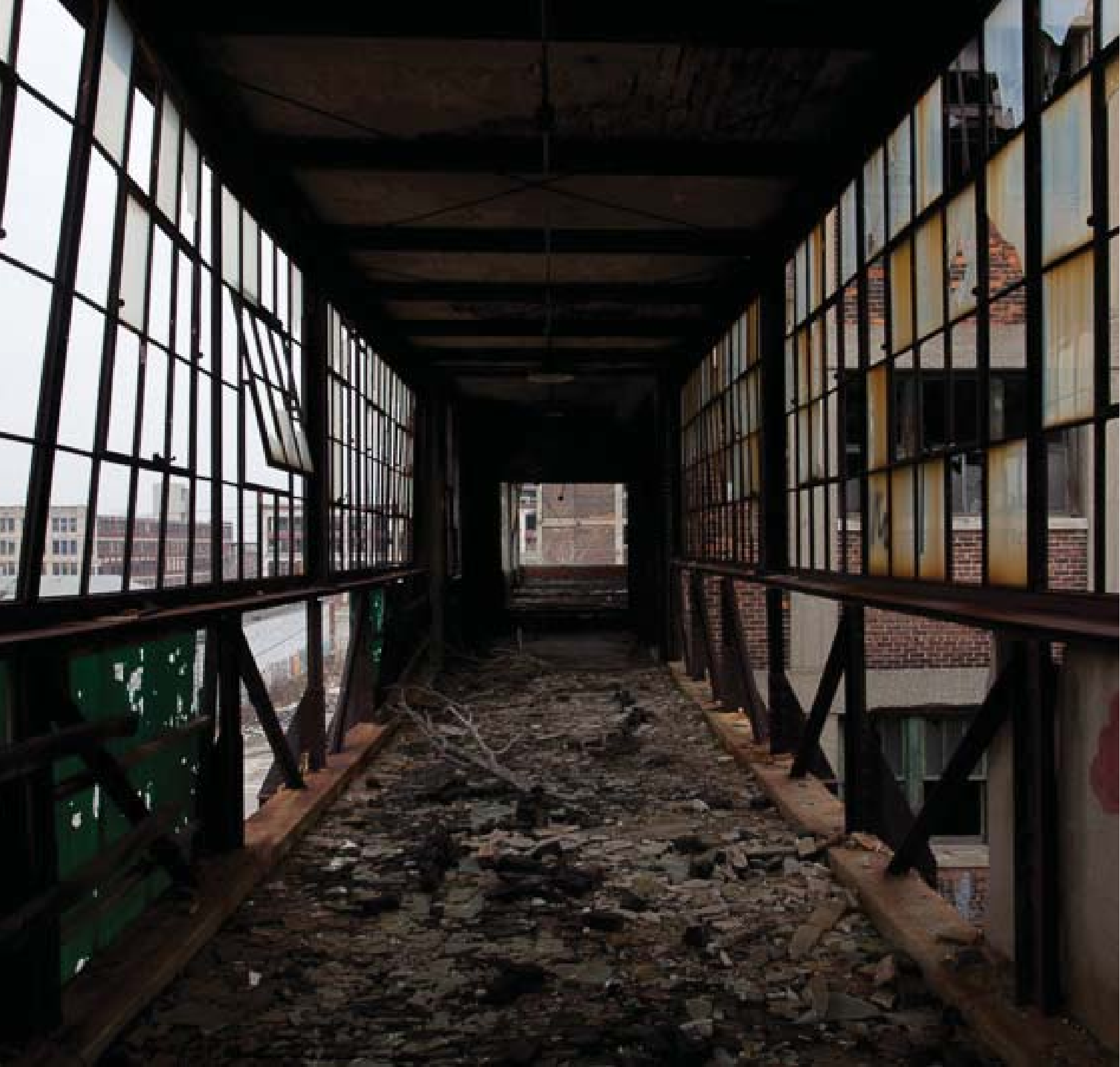
[42] (Left) Pedestrian bridges once linked buildings within the complex.
