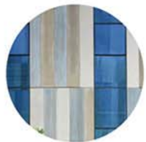
2 Facade / Inner Street 幕墙/内街
