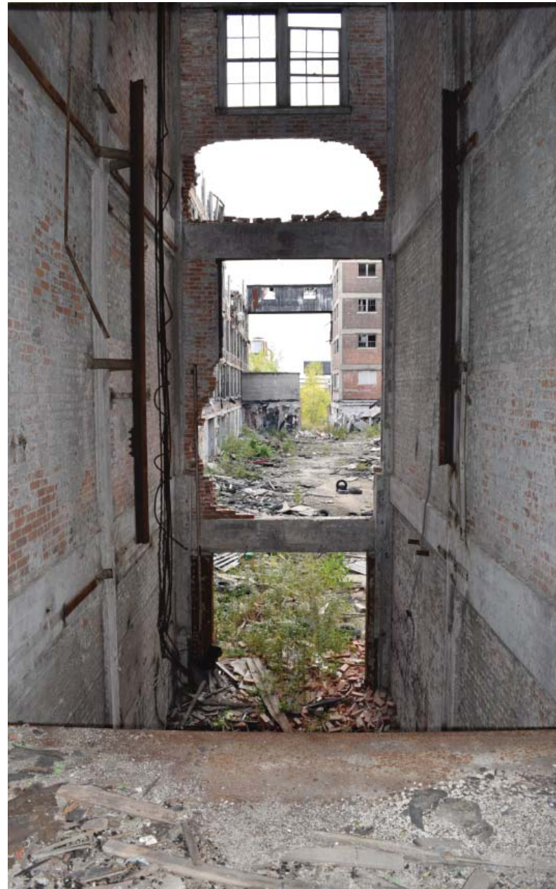
[46] Abandoned elevator shaft.
