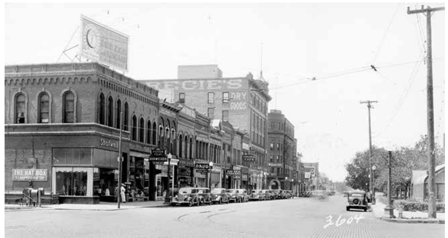
Front Street Looking West in 1930
