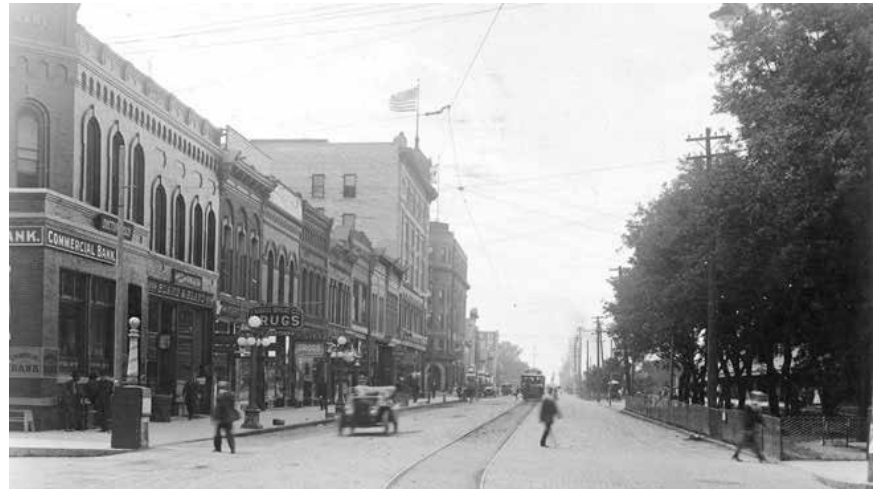
Front Street Looking West in 1910
