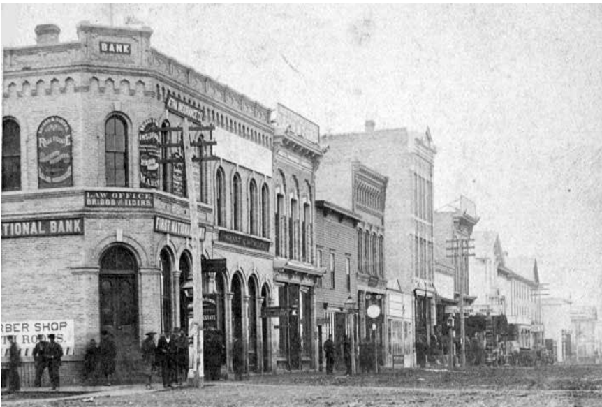
Front Street Looking West in 1879
