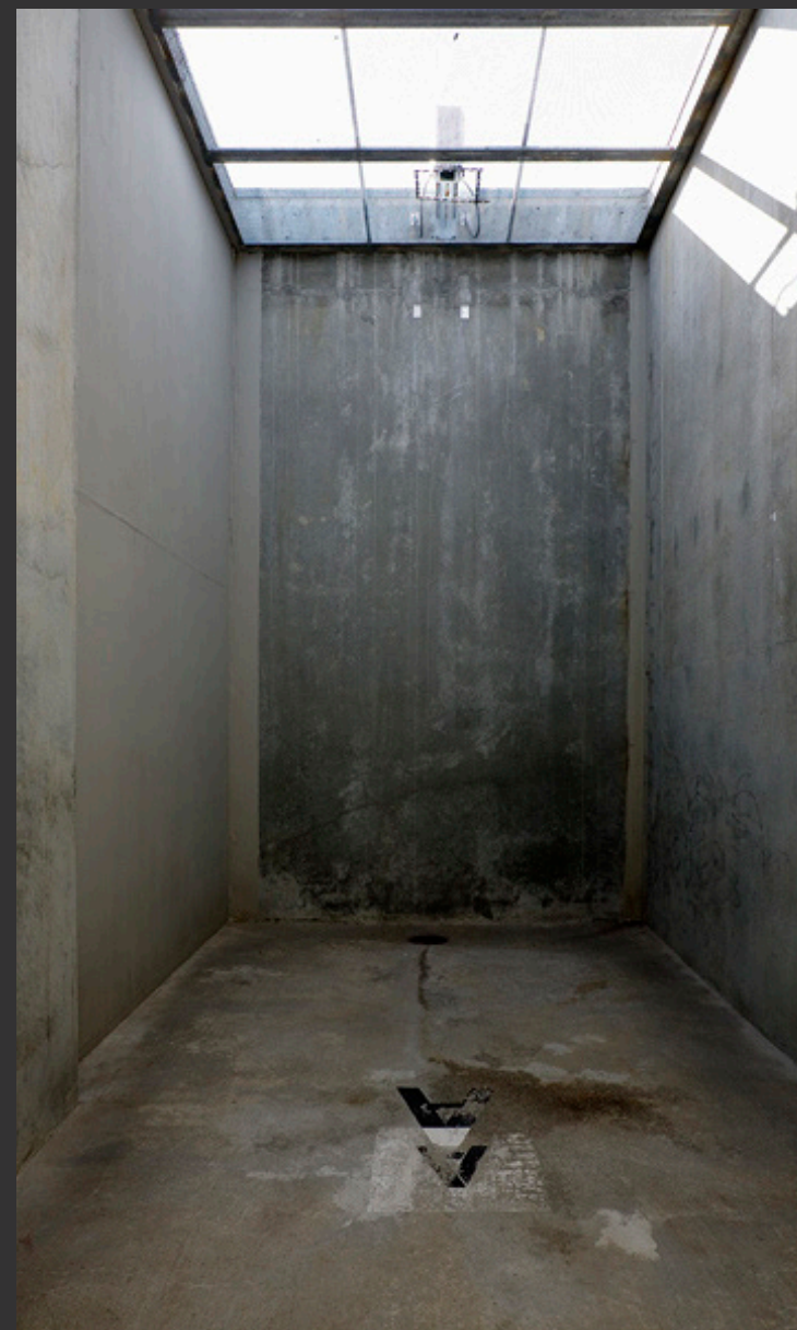
FIG. 050 - PELICAN BAY SOLITARY EXERCISE YARD
