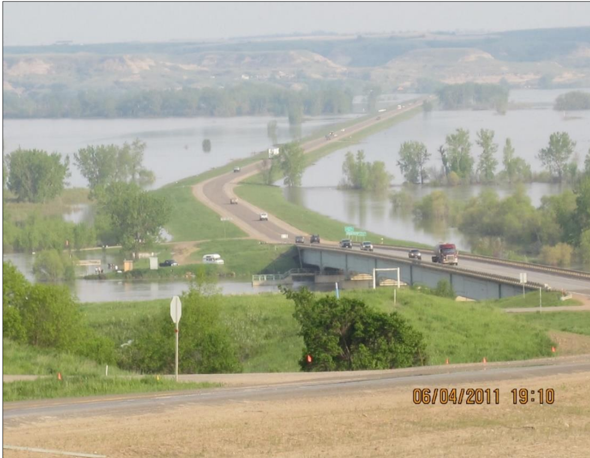
Fig. 96. Flooding of the Missouri River, summer 2011 Highway 85 west of Williston, ND
