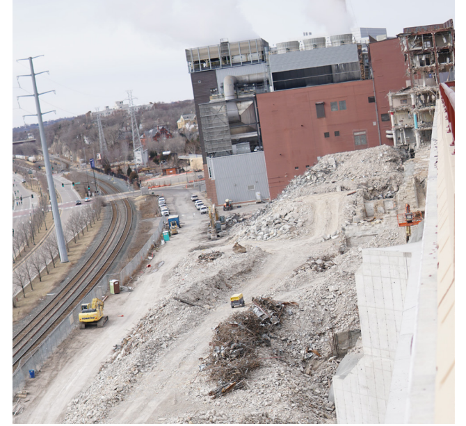
Demolition on site location
