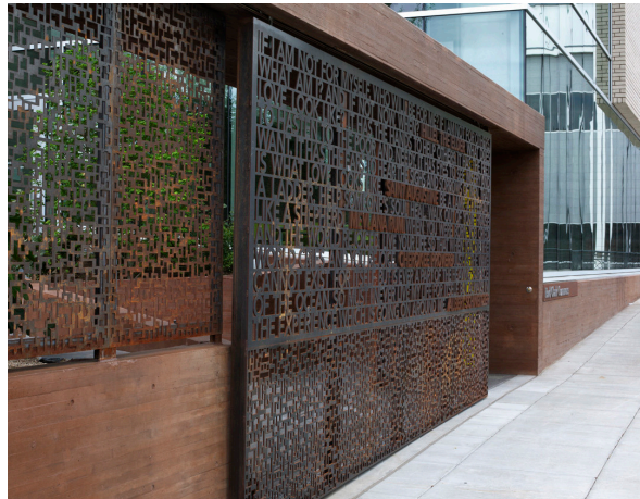
Entrance door. Fig. 17
