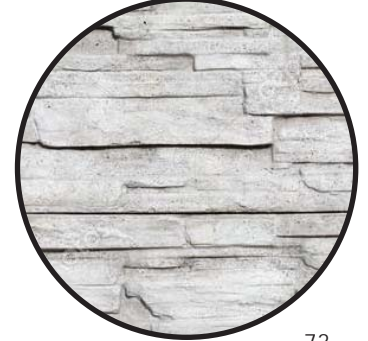
board formed concrete 73
