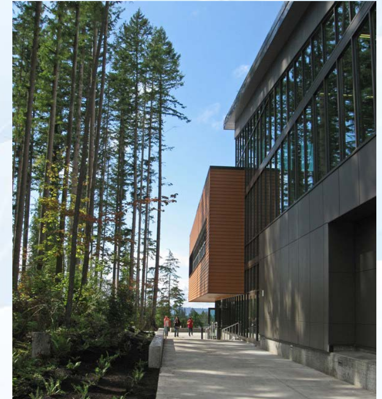
Figure: 20 Item: Marysville Getchell Exterior Perspective Retrieved At: http://www.archdaily.com/155917/marysville-getchell-high-school-
