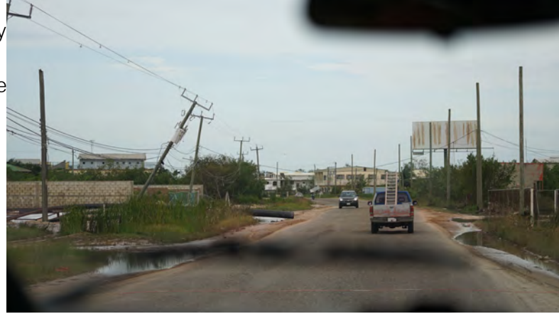
FIGURE 1: CONDITIONS AFTER THE HURRICANE DELT ITS DAMAGE.
