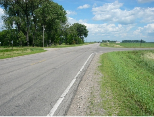
Radius treatment, viewed from west approach.
