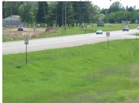
Exclusive lane treatment, east approach in view.
