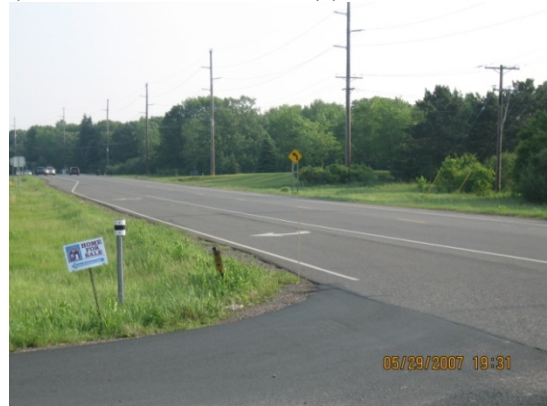
Exclusive lane treatment, north approach in view.
