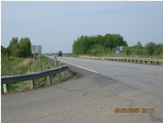
Radius treatment, east approach in view.
