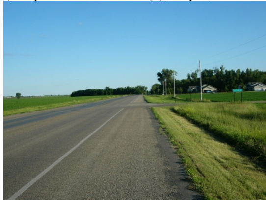
Radius treatment, viewed from north approach.
