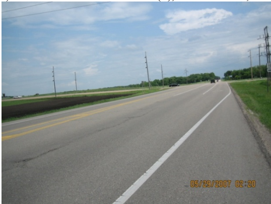
Exclusive lane treatment, viewed from west approach.
