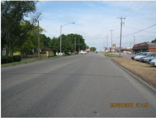
Radius treatment, viewed from east approach.
