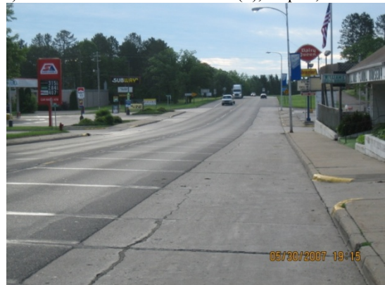
Radius treatment, viewed from west approach; also shows intersecting 11 th St. NE and Subway-DQ driveways.
