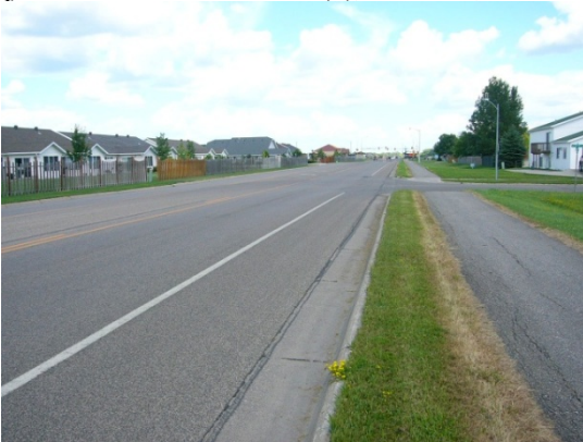
Radius treatment, viewed from west approach.
