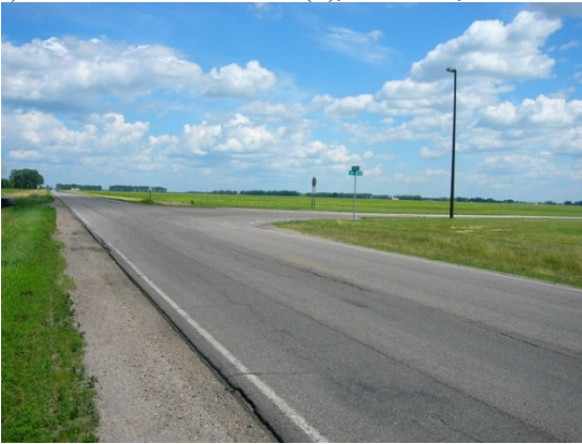
Radius treatment, viewed from west approach.
