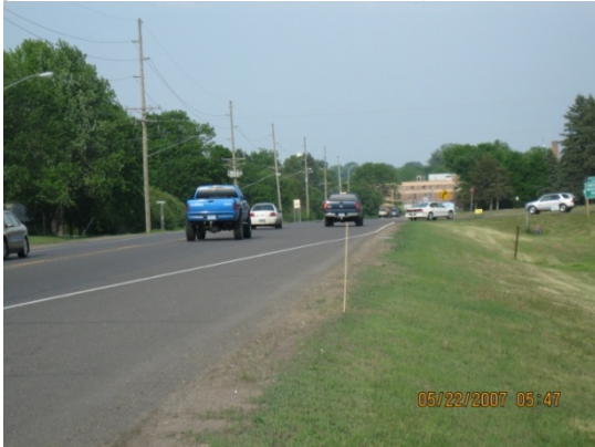
Exclusive lane treatment, viewed from west approach.
