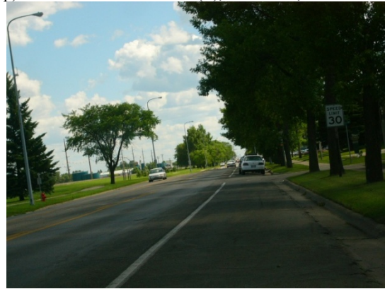
Radius treatment, viewed from north approach.
