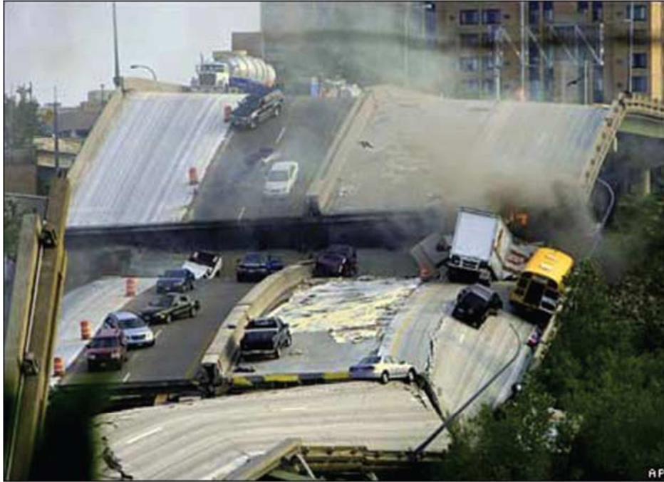
Figure 1.1. The collapsed I-35W bridge with vehicles on. With permission from [4]. Copyright 2007, USFA.
