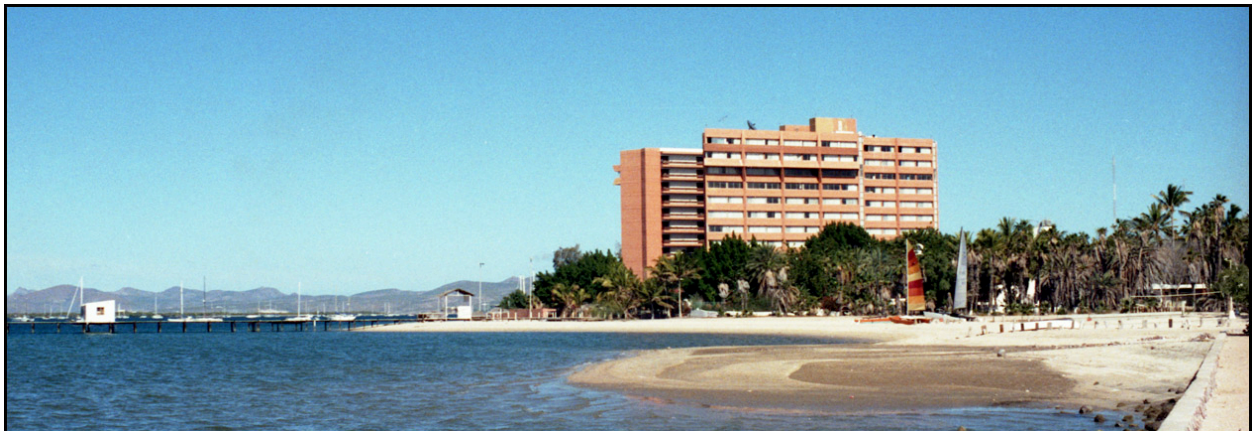
Figure 13. Hotel Gran Baja (The grounds of the Hotel Posada are visible to the right, with small boats beached there. The pier to the left with the white structure at its end is where I fished, the day I first observed the two hotels).
