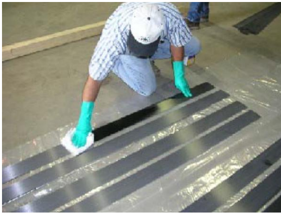
(c) Cleaning and epoxy application on CFRP
