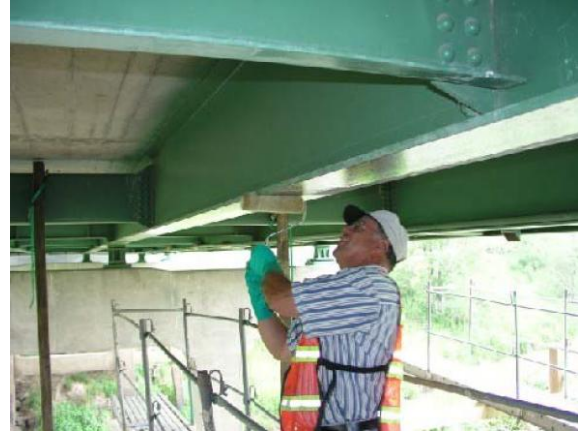
(b) Surface preparation
