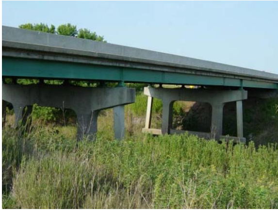
(a) Side view of bridge
