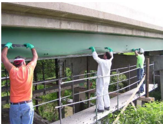
(e) Installation of CFRP plate on beam
