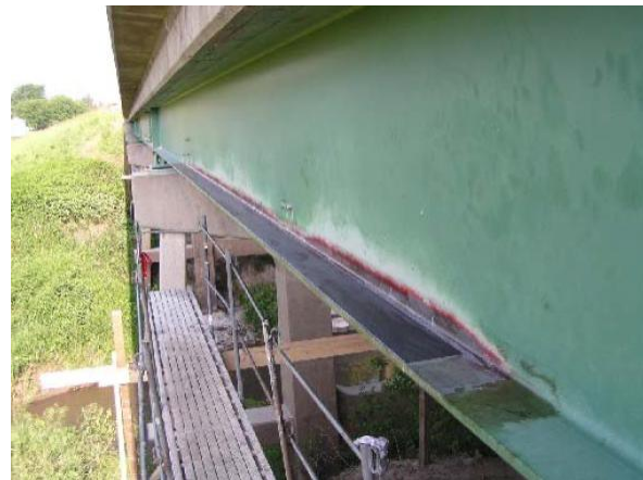
(f) Installed CFRP plate
