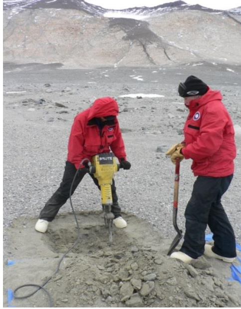
Figure 4.1. Pit Excavation. Pits were excavated using hand tools until reaching ice-cemented (frozen) sediments. Below the frost line, a jackhammer and portable generator were used to excavate the pits to the alluvial-till contact. Photograph courtesy of Adam Lewis.
