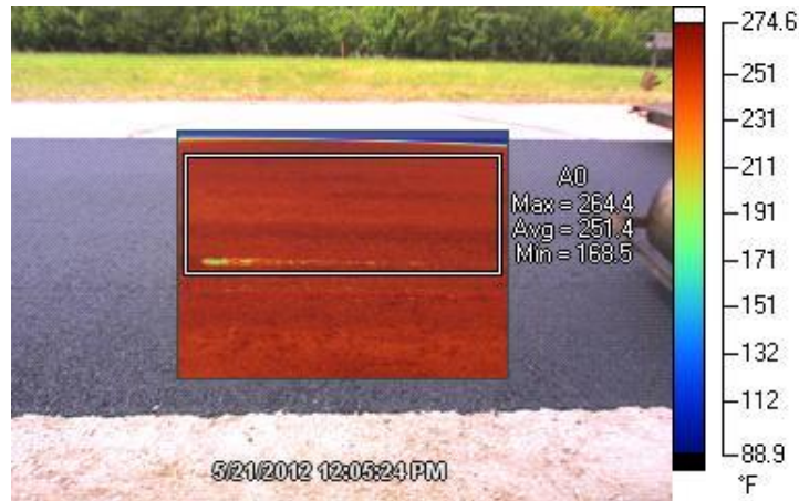
Figure 6. Sample picture of asphalt mat temperatures (Song and Gao, 2012)
