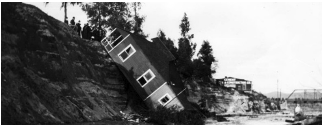
Figure 7. The devastating damage done by the floods in the 1930s.
