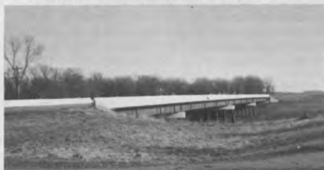
New bridge over Wild Rice River east of Hendrum, built in 1978.
