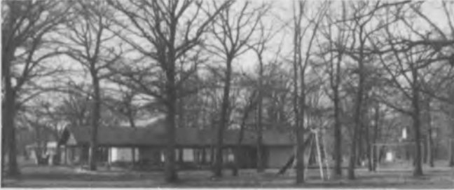
Hendrum Park, View of open air shelter built in 1978.
