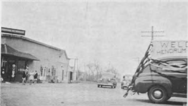
Taken in the 1930's — Note the former State Bank has been converted into a Standard Station. Behind the station the former Ingberg Grocery Store.
