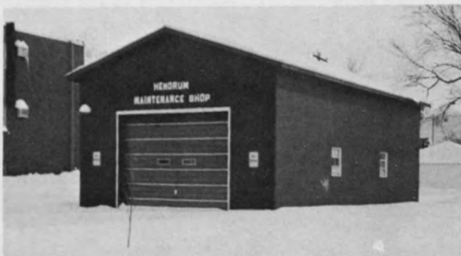
Hendrum Maintenance Shop, the former Norman Highway Dept.
