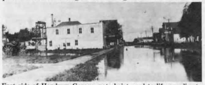
East side of Hendrum Garage, note hoist used to life supplies to upper floor. There was once a ramp leading to top floor. To lower left are steps into the Mission House.
