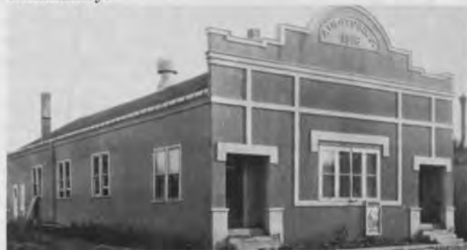
Auditorium, Hendrum, Minnesota
