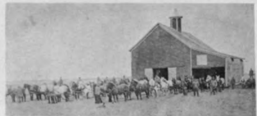
James A. Johnson moving a building with horses. Johnson is grandfather of Harry and Duane Johnson.
