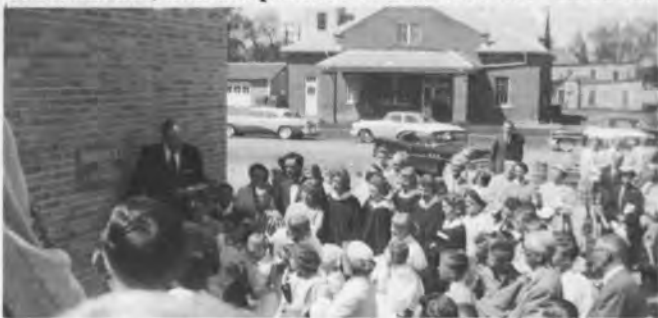
Laying of the Cornerstone, Sunday, May 25, 1958
