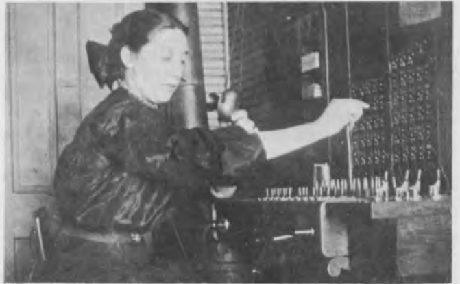
1909-1911 Hendrum Telephone Office. Bessie Hagen Ohnstad at switchboard.
