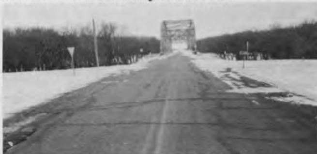
Red River Steel Bridge, built in 1950, an extension in 1970.
