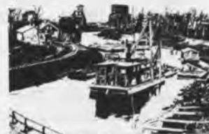
Red River as seen from the N.P. Bridge
