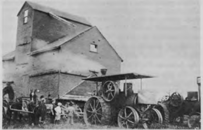
James A. Johnson moving the elevator from Hendrum to the Dick Canning farm with steam engines, 1908.
