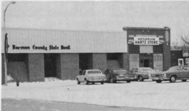
Norman County State Bank, after remodeling in 1975.
