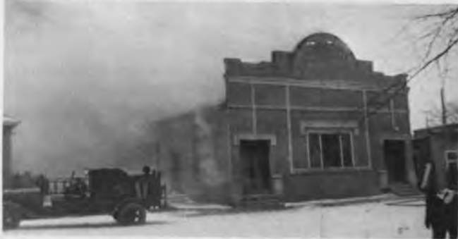
Auditorium destroyed by fire, 11-23-50 As photographed by Irving Storsved
