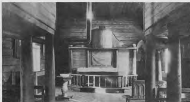
Interior of old Hendrum Church
