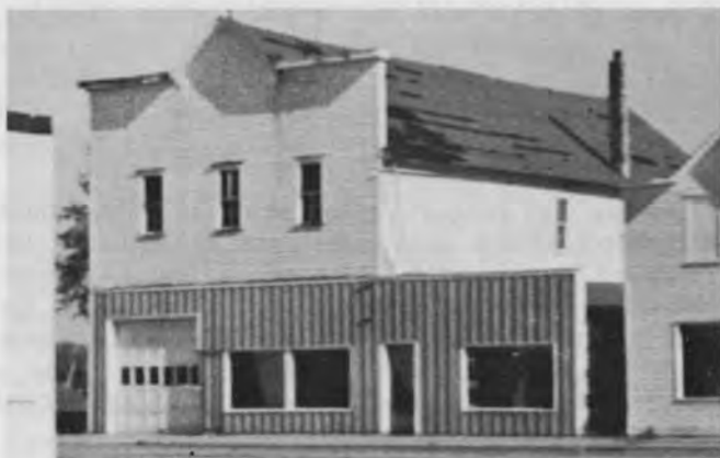
Ostenson Motor Sales and Service, center high building.
