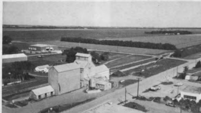
Hendrum, 1980. Taken from water tank, northwest direction. Farmer's Elevator, Hendrum Manufacturing, Mobil Oil.
