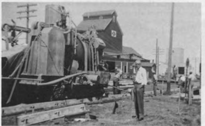
Laying the pavement through Hendrum in 1954. Art Hansen.
