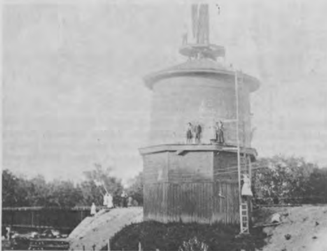
Great Northern water tank north of Hendrum
