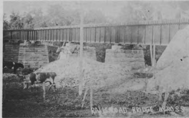
Railroad bridge across Wild Rice, north of Hendrum
