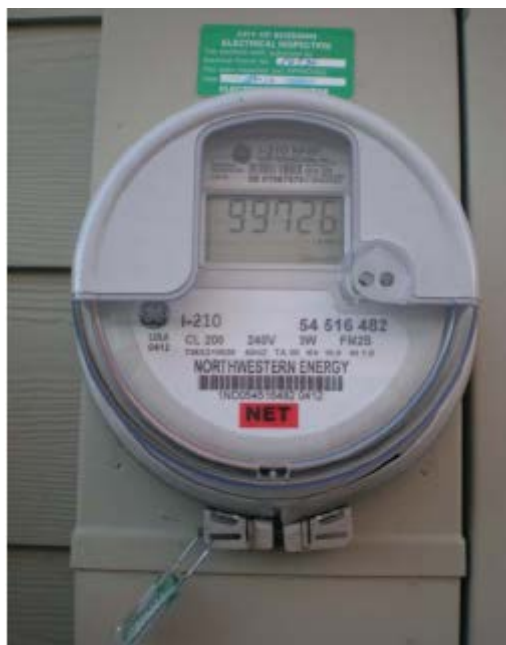
Figure 1.1. A smart meter. Photo sourced from National Renewable Energy Laboratory (NREL) database, PIX 21394, http://www.osti.gov/bridge .
