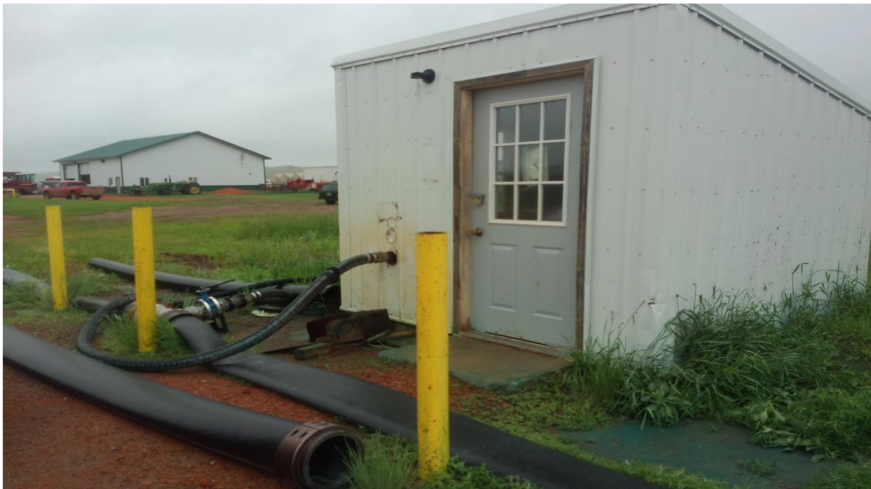
Figure 3. Water Depot. Source: Tong Lin (NDSU).
